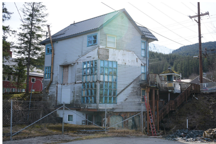
Image left: Rehabilitation project. Photo credit: Forrest Courtney
