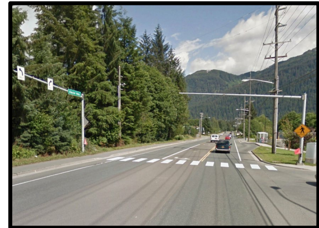
Uncontrolled crosswalk on Glacier Highway (Source: Google Earth)
