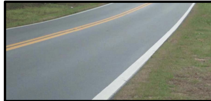
Wider (6 inch) edge lines (Source: FHA)
