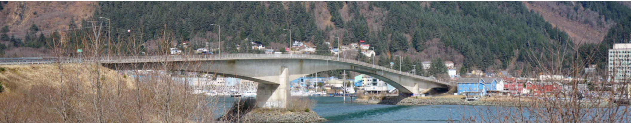
Image: Douglas Island Bridge. Photo credit: Forrest Courtney.
