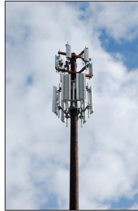
Sectorized (panel) Antenna Array
