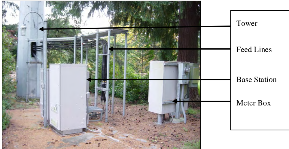
Figure 1: Example of 1900 MHz Wireless Infrastructure Ground Equipment
