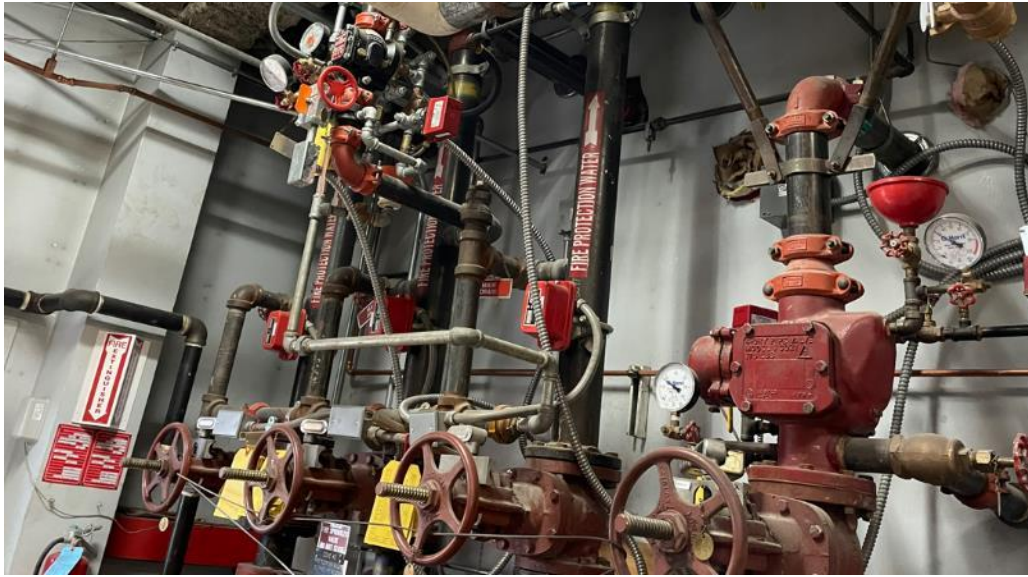
Fire sprinkler system risers for the terminal
