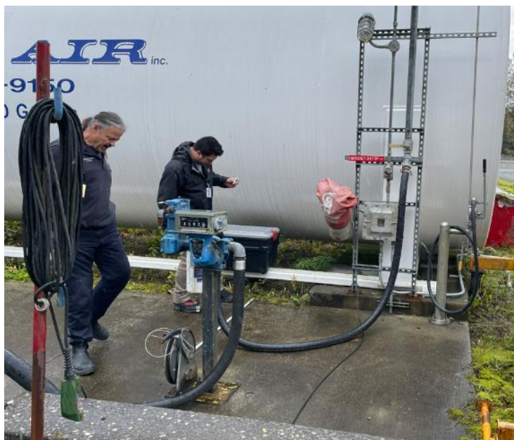
Ward Air mobile fueler filling station (left) and emergency fuel shut-off valve within the probable spill zone
