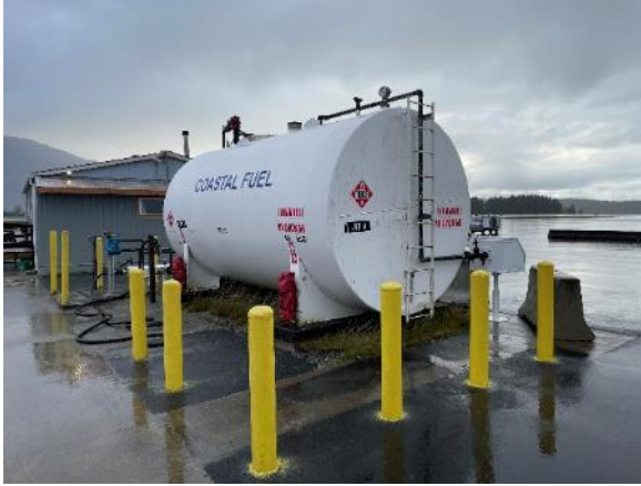
Coastal Fuel Jet A fuel tank, highly visible placards, but no bonding cable, deadman control, or overfill protection system
