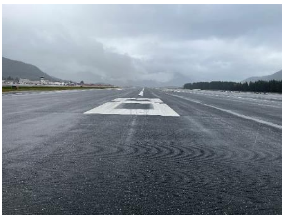
Runway 8 designator and in-pavement center line lighting
