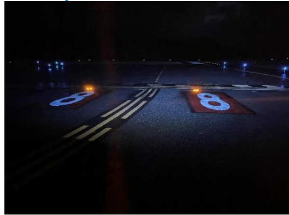
Taxiway B surface painted hold position markings and enhanced taxiway markings
