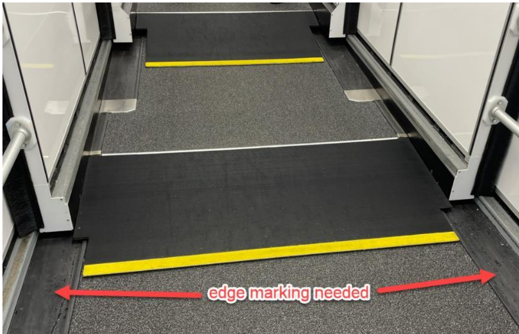
New Gate 5 Jetbridge needs edge markings for uneven surfaces
