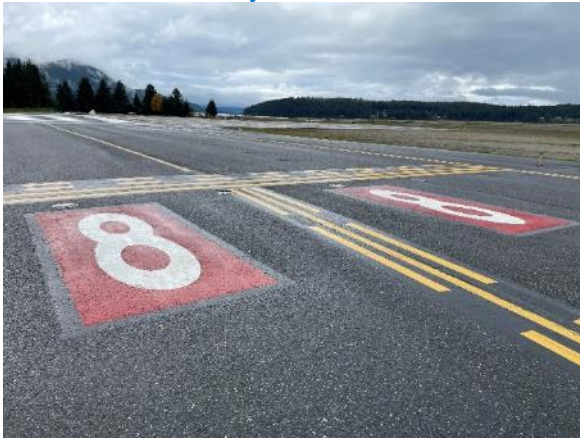
Taxiway B surface painted hold position markings and enhanced taxiway markings
