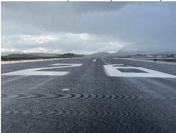
Runway 26 designator and in-pavement center line lighting
