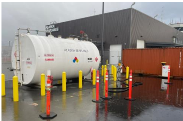
Alaska Seaplanes newly relocated Jet A fuel tank for supplying mobile fuelers
