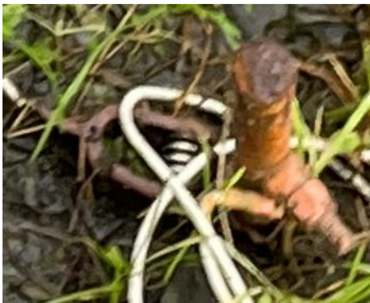
The bonding cable was clipped to a ground post
