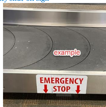
New warning baggage belt warning placards and emergency shut-off sign
