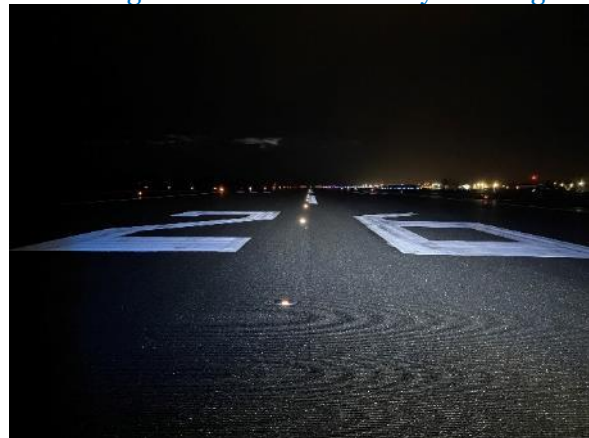
Runway 26 designator and in-pavement center line lighting
