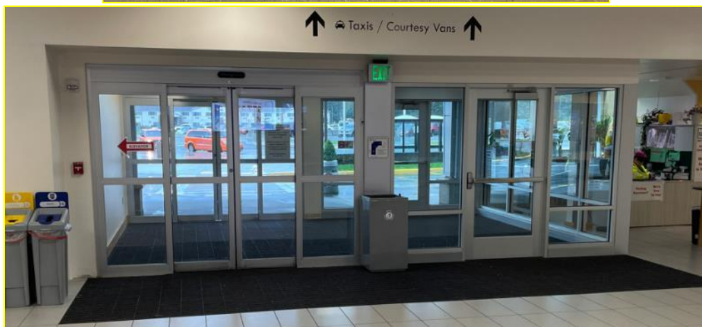
All vestibules have in-ground walk-off mats, flush with the tile surface with no exposed edges
