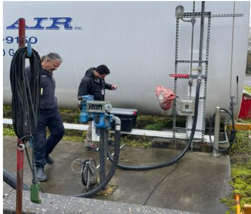
Ward Air emergency fuel shut-off well within the probable spill area (left) and defective bonding cable clip (right)
