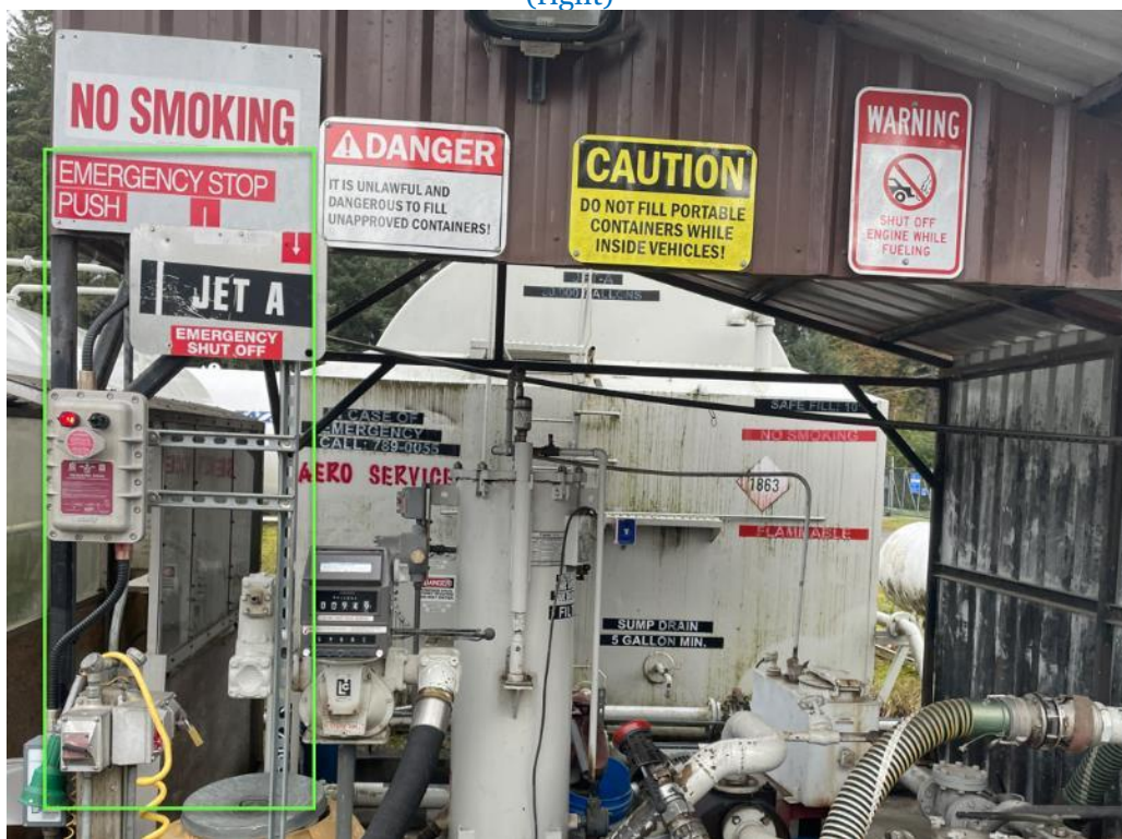
Aero Services fueling station with confusing and inaccurate placarding
