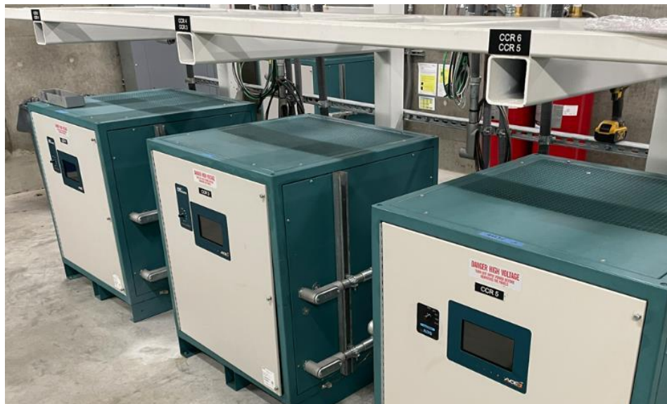
Primary vault regulators with circuit names (CCR 5, CCR 6, etc) on black placards, but with no other references
