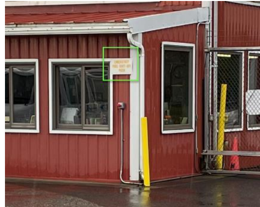
Ward Air emergency shut off valve is located outside of the “probable spill area”, but the placard is faded and should be replaced
