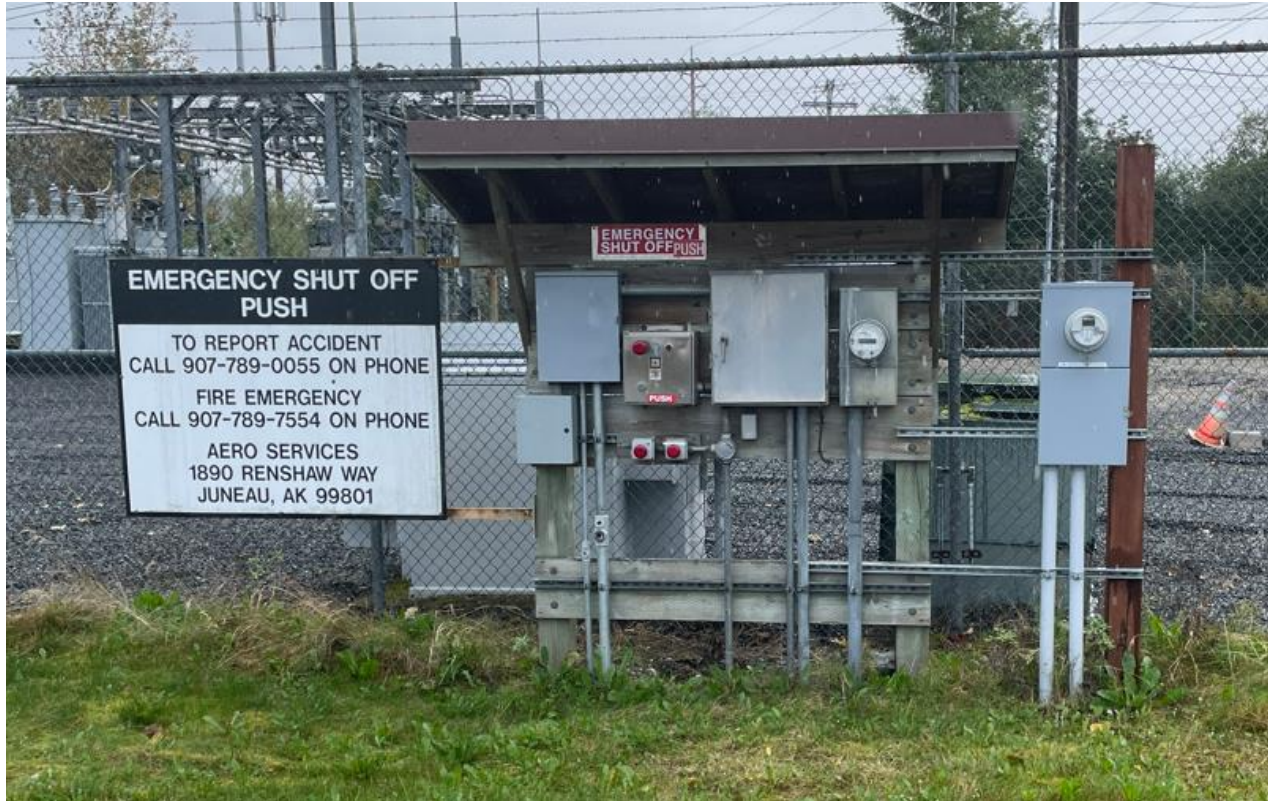
Remote emergency fuel shut-off station with multiple push buttons without explanation
