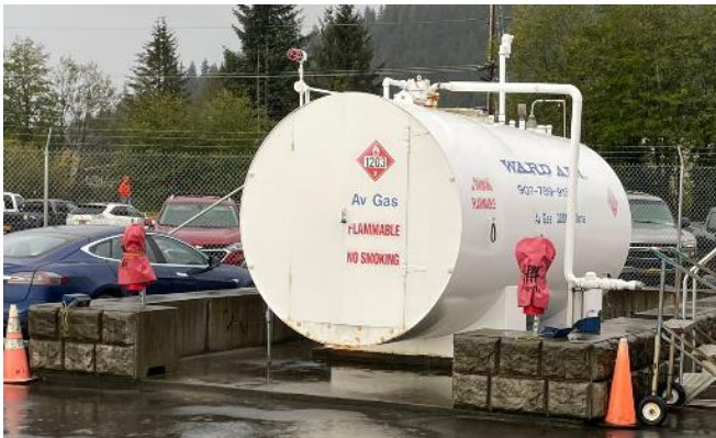
Ward Air airfield based Av Gas supply tank (left) and faded and illegible emergency fuel shut-off sign (right)
