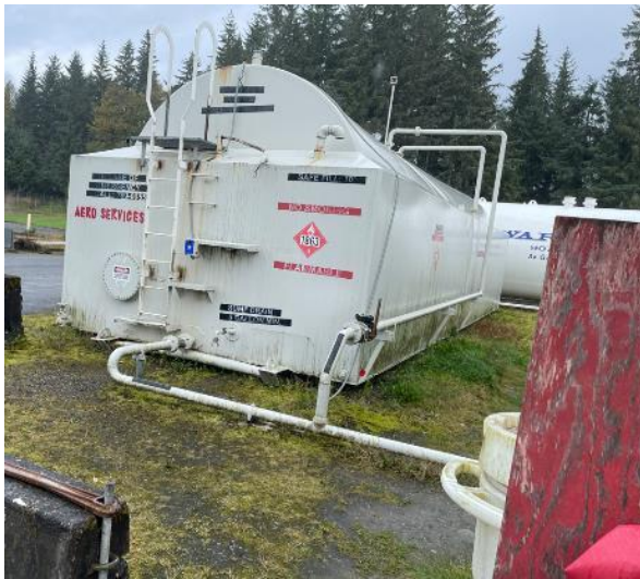
Aero Service fueling station with two Jet A tanks, which lacks vehicle impact protection to the fuel control station (right)
