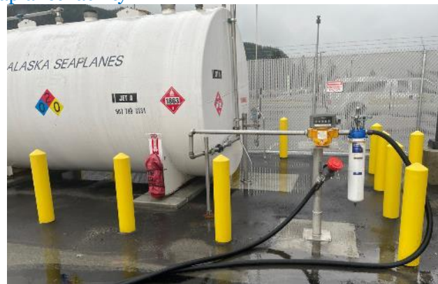
Alaska Seaplanes newly relocated Jet A fuel tank for supplying mobile fuelers
