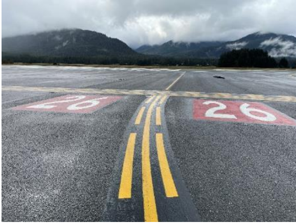
Taxiway G surface painted hold position markings and enhanced taxiway markings
