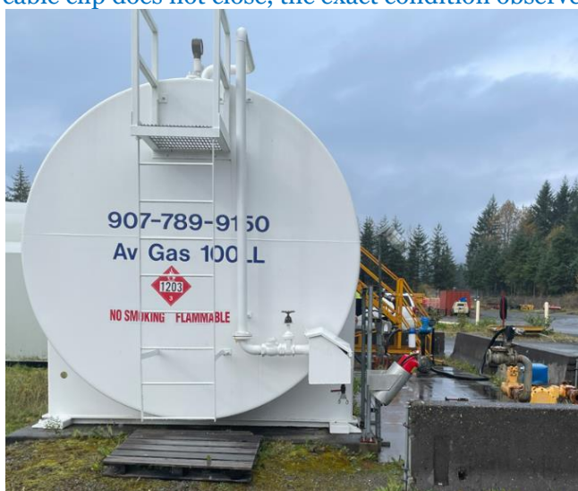
Ward Air supply tank intake for filling, no deadman or overfill controls
