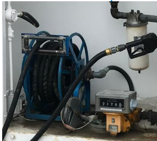
The fuel tank filling equipment contains safety features include bonding cable and deadman control
