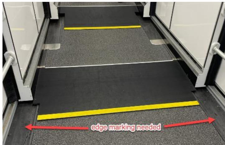
New Gate 5 Jetbridge needs overhead and edge markings for uneven surfaces
