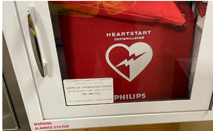
AED cabinets located throughout the terminal, no label indicating date of last service
