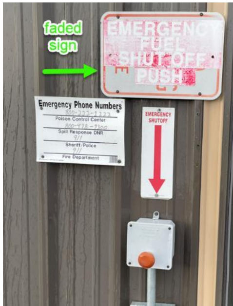
Emergency fuel shut-off station on the wall of the hangar with faded sign (left) and NFPA 407 section on placarding (right)
