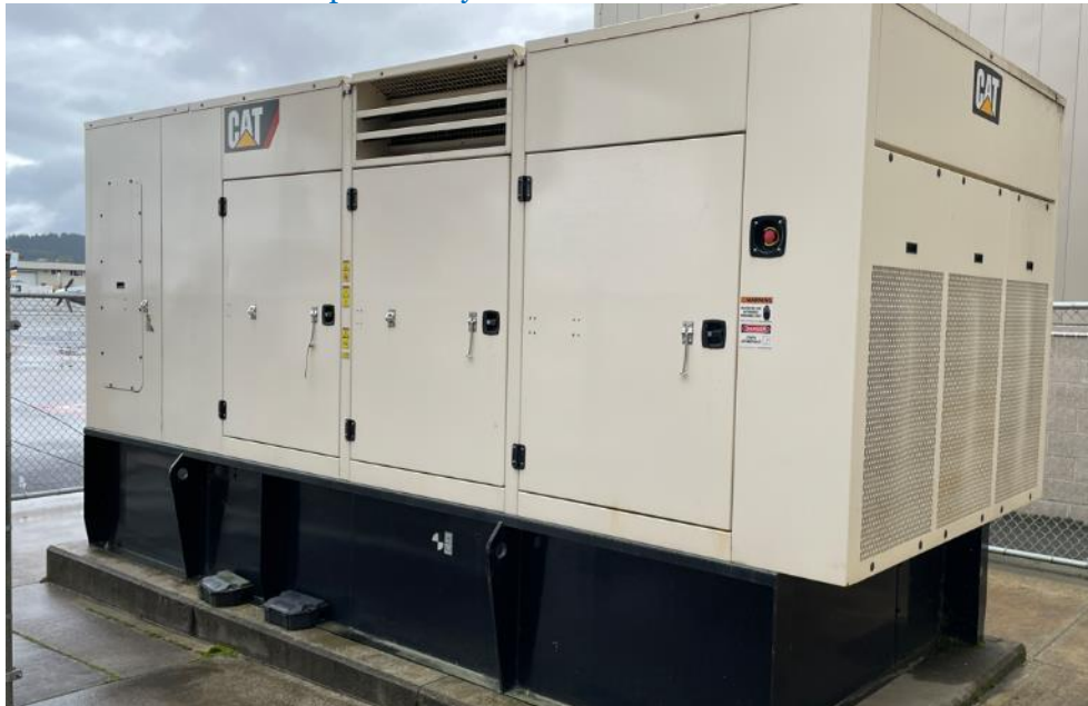
Diesel generator for critical electrical systems in the terminal
