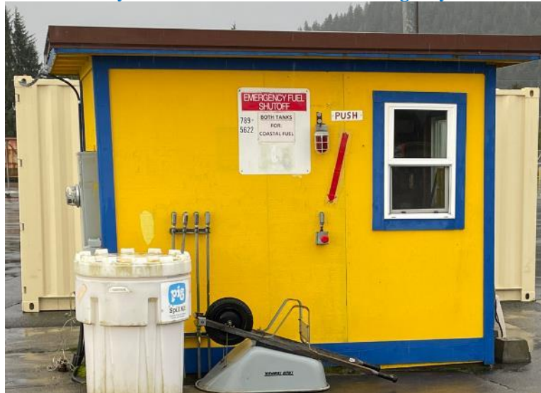
Coastal fuel tank and yellow hut with the emergency fuel shut-off station
