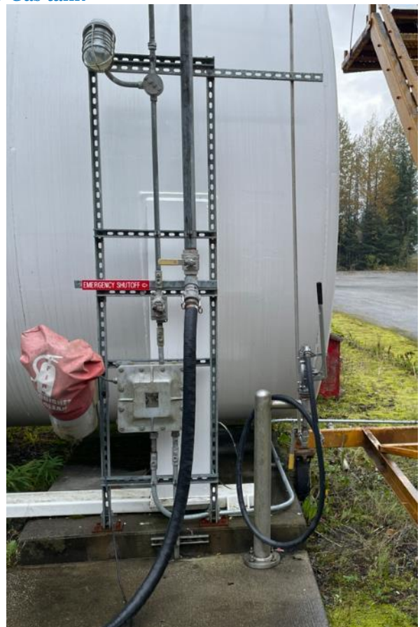
Ward Air mobile fueler filling station (left) and emergency fuel shut-off valve within the probable spill zone
