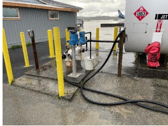
Coastal Fuel Jet A fuel tank, highly visible placards, but no bonding cable, deadman control, or overfill protection system
