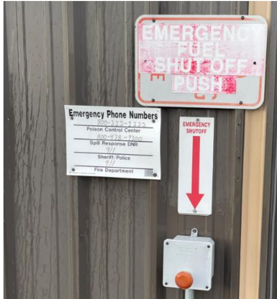
Faded placard to be replaced and installed at seven feet above ground
