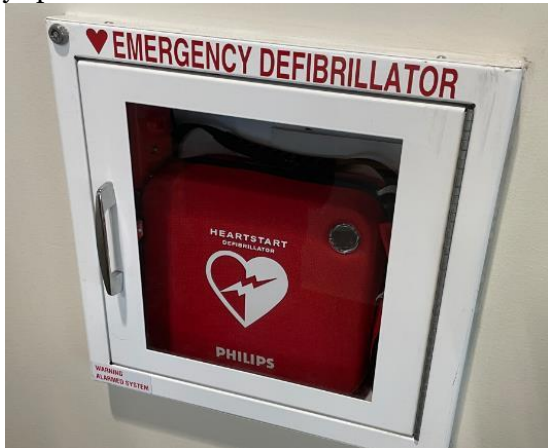
AED cabinets located throughout the terminal, no label indicating date of last service
