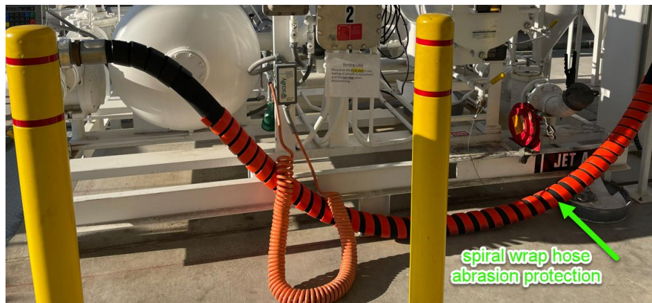
Example of a hose protected in plastic spiral wrap to mitigate degradation from surface abrasion
