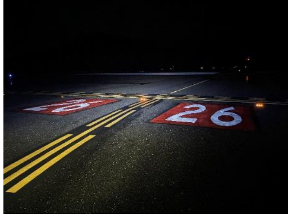
Taxiway G surface painted hold position markings and enhanced taxiway markings
