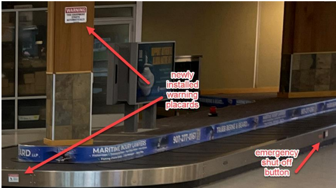
New warning baggage belt warning placards and emergency shut-off sign
