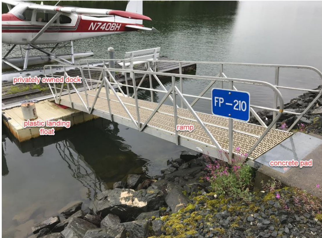
Components of a leased float pond dock
