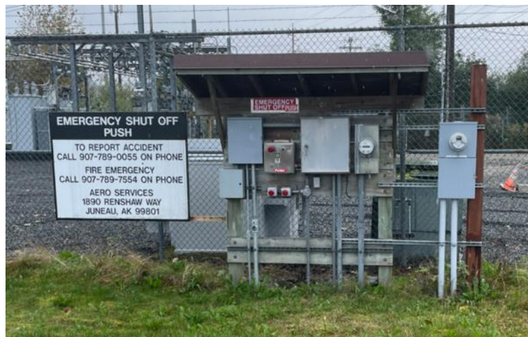
This should be configured to be the sole emergency fuel shut-off station for Aero Services and Ward Air fuel farm tanks (if approved by the Fire Marshal)
