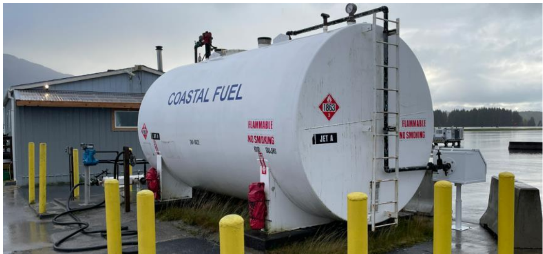
Coastal Fuel airfield based Jet A supply tank
