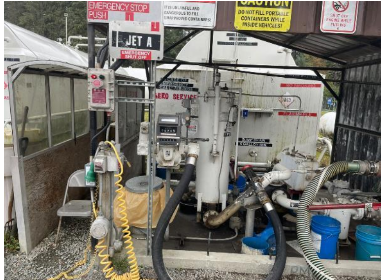
Aero Service fueling station with two Jet A tanks, which lacks vehicle impact protection to the fuel control station (right)
