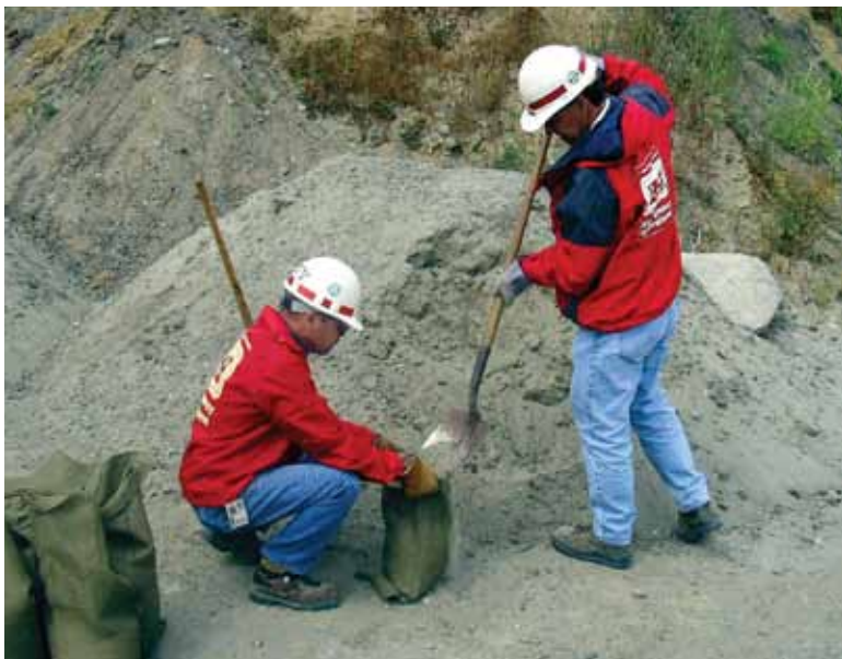
This two-member team uses proper techniques for sandbag filling.
