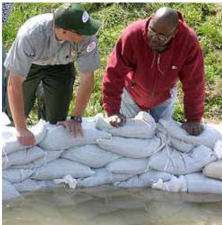
Engineers inspect placement of sandbags
