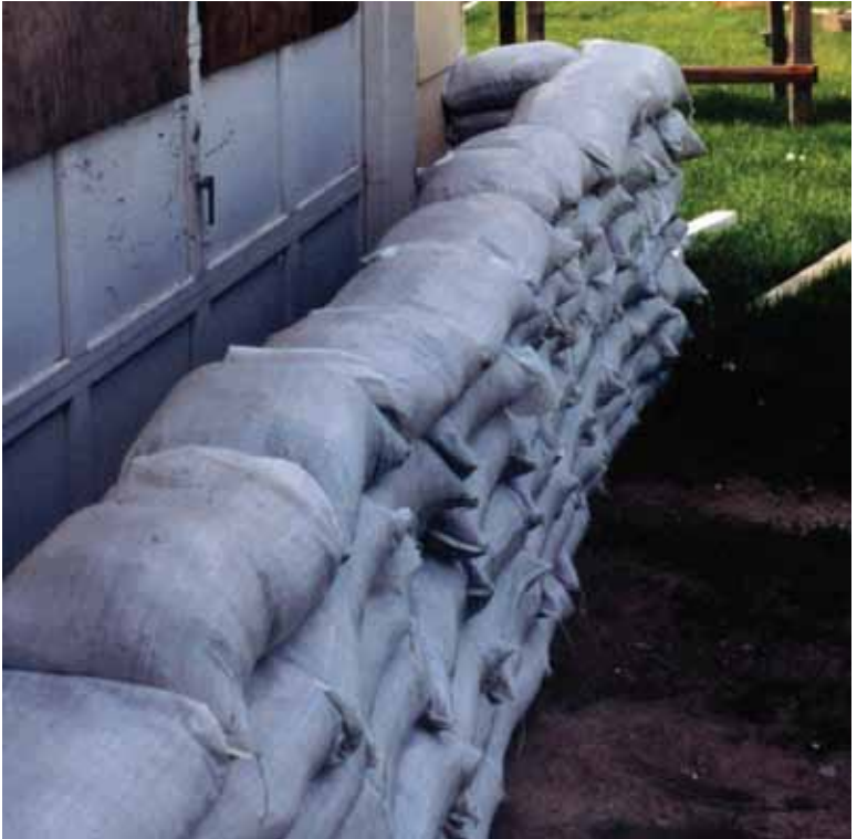
Single stack placement
