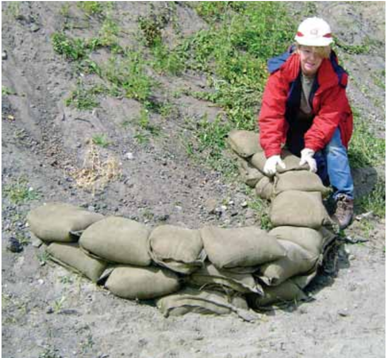
A Corps employee demonstrates building a ring dike.
