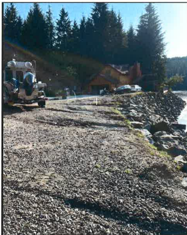
Image #3: Minor Erosion of bank along Rivercourt Drive from flood water draining back into the river
