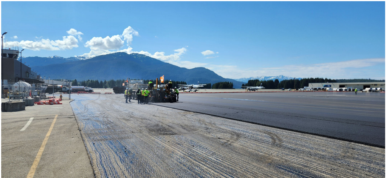
Photos above and below: SECON paving the top lift of asphalt paving within the Phase 8 and Phase 10 (north end of the 135 apron) work areas.
