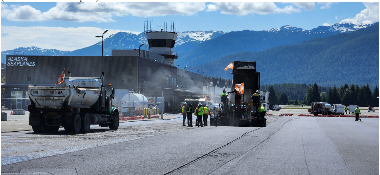
Photos above and below: SECON paving the top lift of asphalt paving within the Phase 8 and Phase 10 (north end of the 135 apron) work areas.
