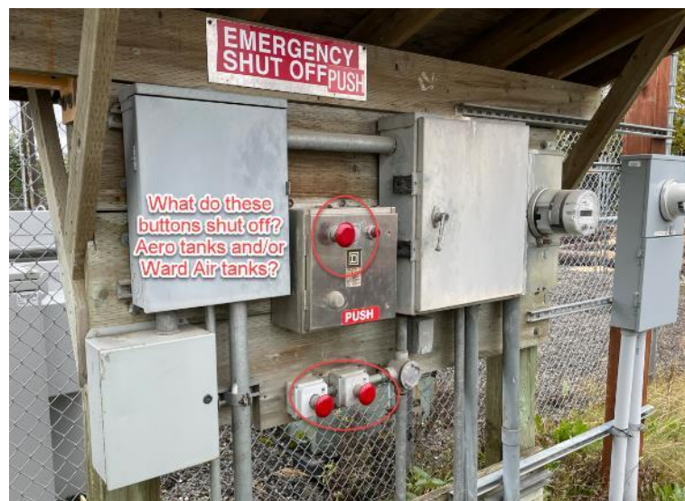
Remote emergency fuel shut-off station at the main fuel farm near the Aero Services fueling station, additional instructional placards needed
