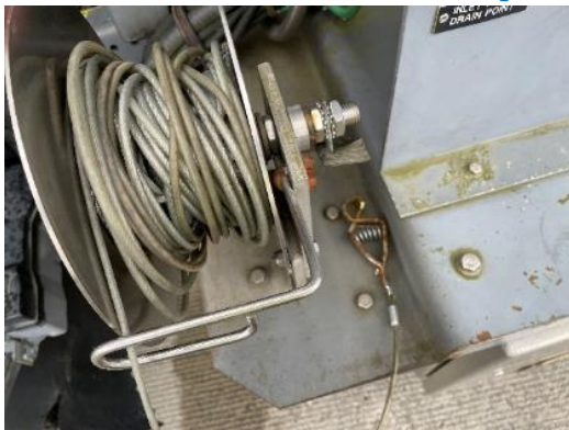
Bonding cable/clip in good condition, the emergency fuel shut-off button is faded and should be painted bright red to restore high visibility appearance
