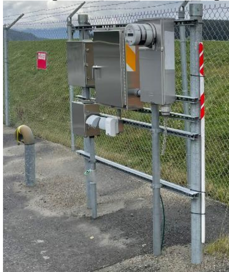
Power hookup panel for the new float pond pump
