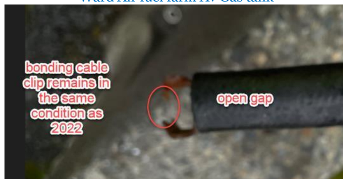
Bonding cable clip does not close
