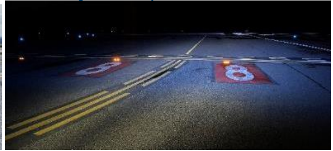
Taxiway B surface painted hold position markings and enhanced taxiway markings
