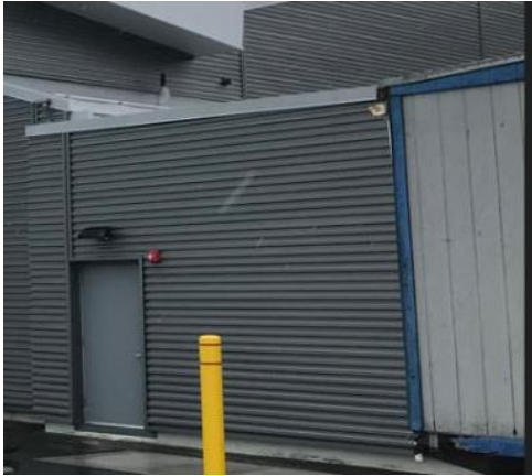
The new airfield lighting electrical vault entrance and interior, Danger/Warning signs needed on the door
