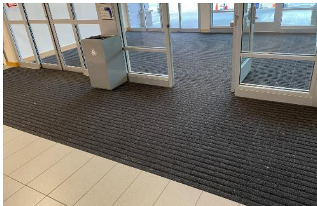
All vestibules have in-ground walk-off mats, flush with the tile surface with no exposed edges
