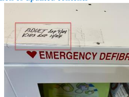
Examples of AED cabinets with tracking of expiration dates of contents
