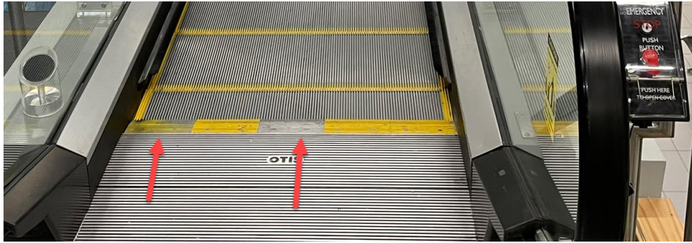
The comb plate of the newer north escalator is missing sections of yellow comb plates on the upper level
