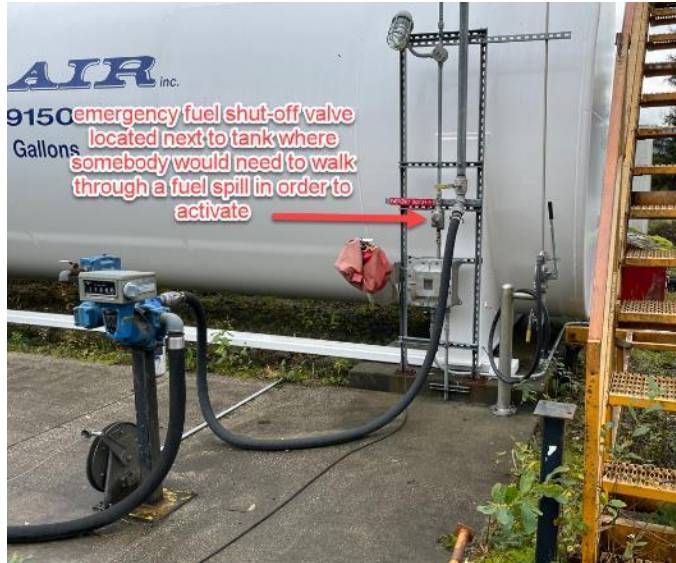
Ward Air Av Gas tank at the main fuel farm, emergency fuel shut-off station located within the probable spill area
