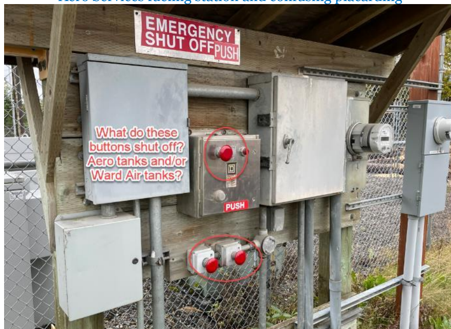
Remote emergency fuel shut-off station
