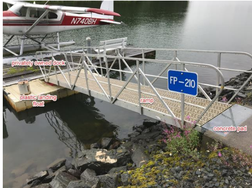
Components of a leased float dock
