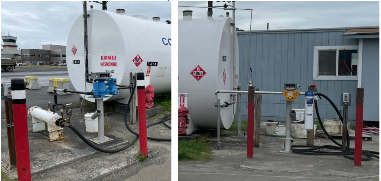
Coastal Fuel (left) & Alaska Seaplanes (right) fueling stations, no overfill protection or bonding cables are present
