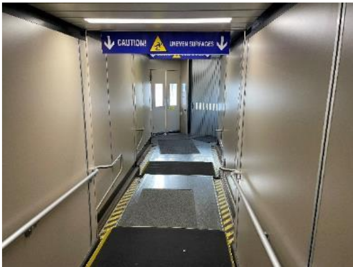
Jetbridge 2 interior, good use of warning signs for surface transitions and edge markings
