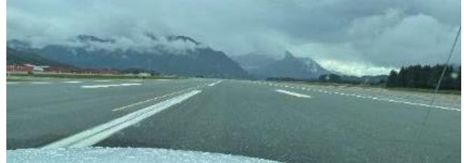
Runway 8 centerline has some rubber build-up, but mostly visible
