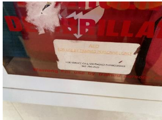
One AED box, no indication of inspection or updated contents
