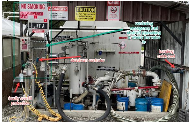
Aero Service fueling station at the main fuel farm, emergency fuel shut-off located within the probable spill area, and the instructional placarding for fuel shut-off should comply with NFPA 407 convention
