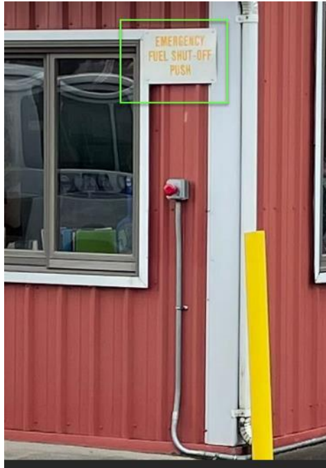
Ward Air faded emergency fuel shut off placard to be replaced
