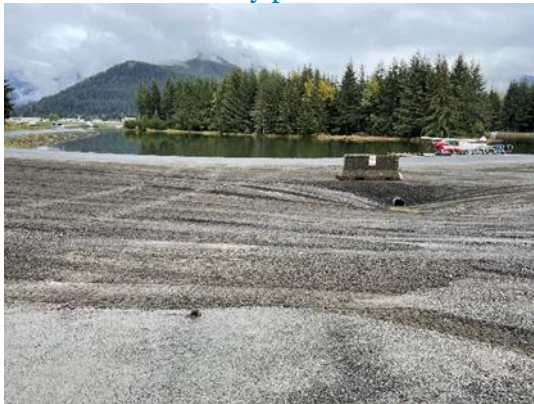
Regraded area with a new culvert
