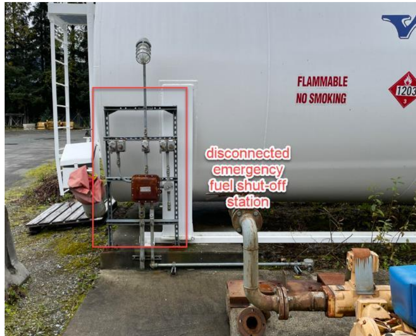
Ward Air fuel farm Av Gas tank, disconnected emergency fuel shut-off apparatus to be removed
