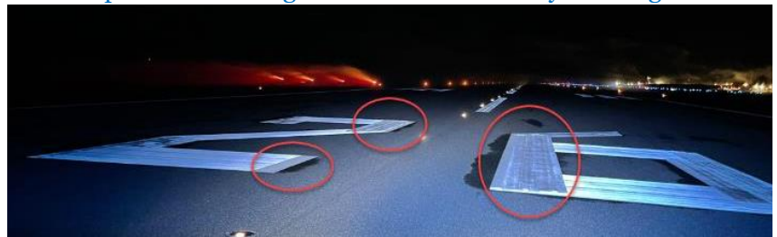
Runway 26 indicator markings also flawed by defective touch up painting. In-pavement center line lighting
