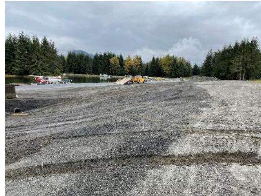
Regraded area with a new culvert
