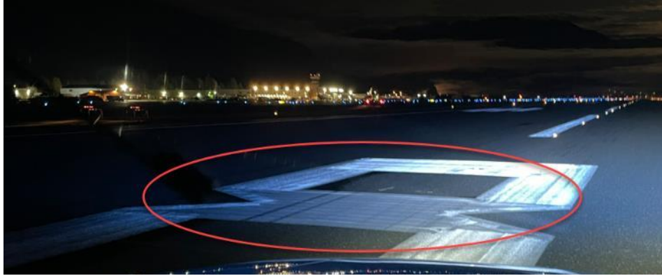
Runway 8 identifier partially flawed reflectivity
