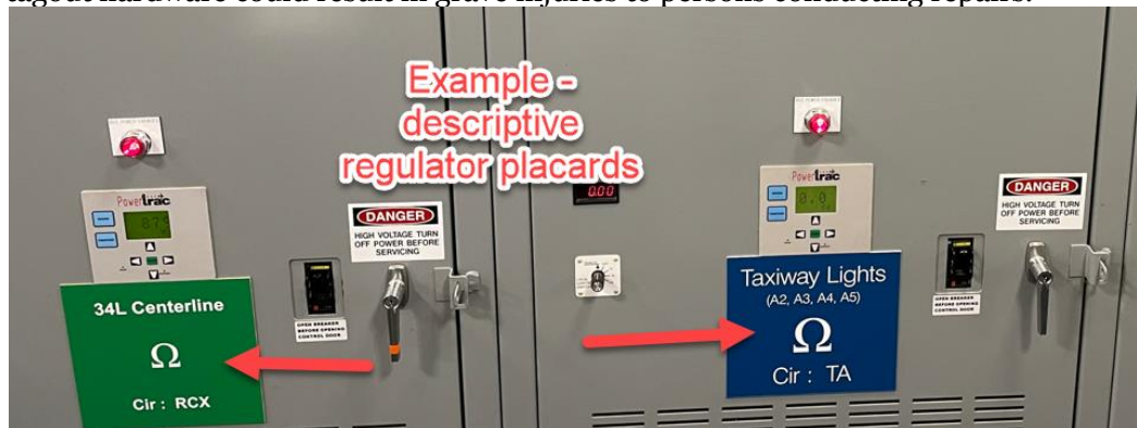
An example of a more definitive airfield lighting regulator placard nomenclature
