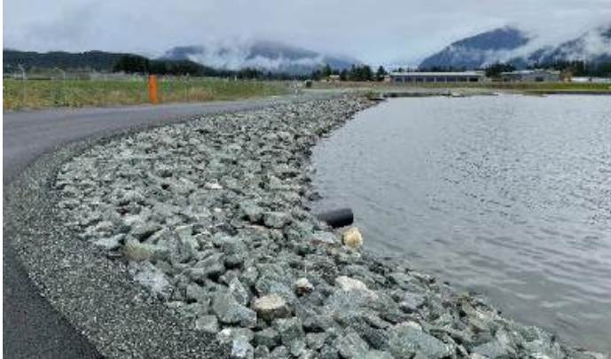
Newly installed rock along the shore, the airport float pond maintenance boat is moored at the dock (right)
