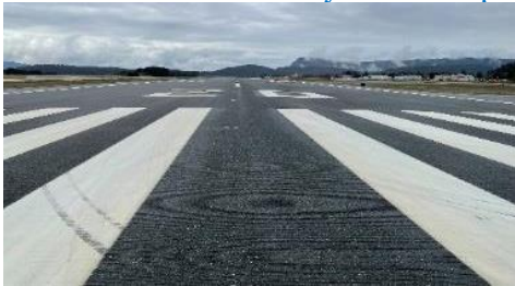
Runway 26 indicator markings also flawed by defective touch up painting. In-pavement center line lighting
