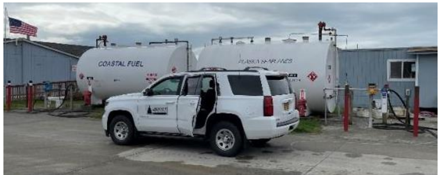
Coastal Fuel & Alaska Seaplanes Jet A fuel tanks, highly visible placards, no bonding cable or overfill protection systems on either tank
