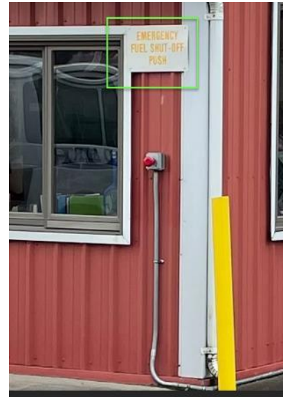
Ward Air emergency shut off valve is properly located outside of the “probable spill area”, but the placard is faded and should be replaced
