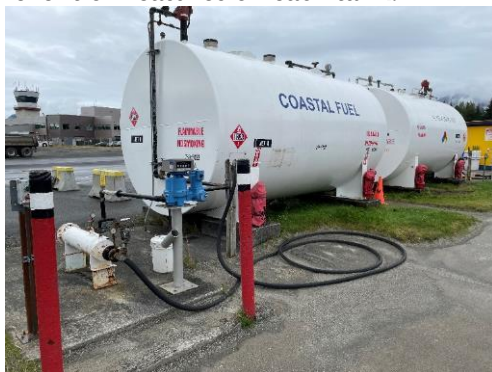
Coastal Fuel & Alaska Seaplanes Jet A fuel tanks, highly visible placards, no bonding cable or overfill protection systems on either tank
