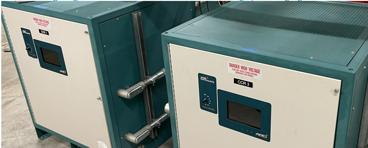
New regulators with circuit names (CCR 1, CCR 3, CCR 9, CCR 10) on black placards, but with no other references
