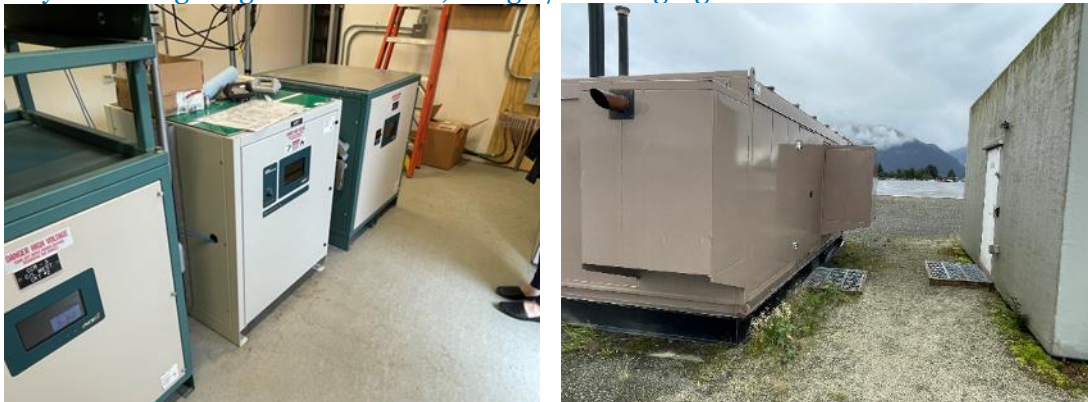
Backup regulators and generator for the old vault
