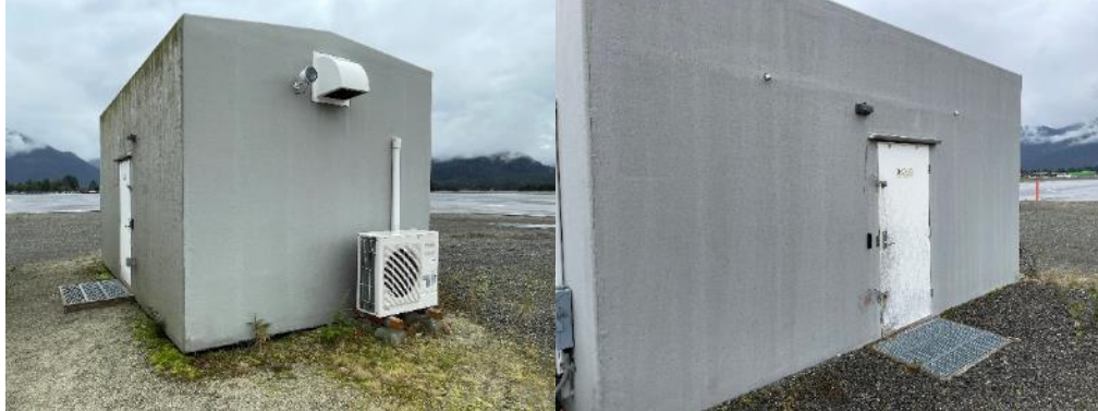
Secondary airfield lighting electrical vault, Danger/Warning signs needed on both doors
