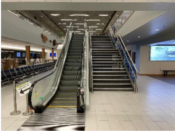
North upward escalator and stairs, the upper end comb plates need consistent yellow coloring across the width
