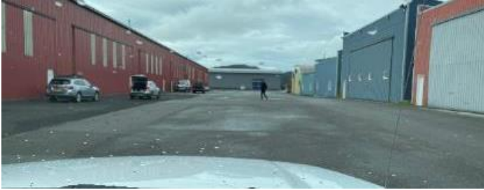
West apron airfield tenant hangars, no center lead-in lines
