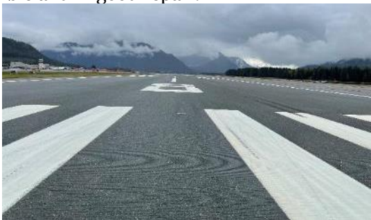
Runway 8 indicator, note center of the “8” glass beads are not reflective due to defective contractor touch up work, in-pavement center line lighting
