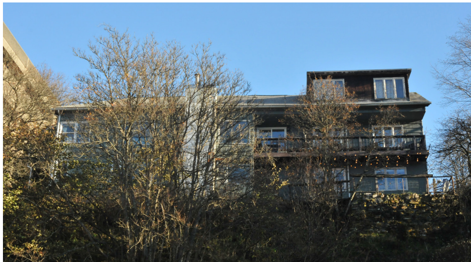
West Facade. Contemporary decks added to allow access to the three basement apartments. The dormer is also a contemporary addition. Peterson-Kasnick House, 2023
