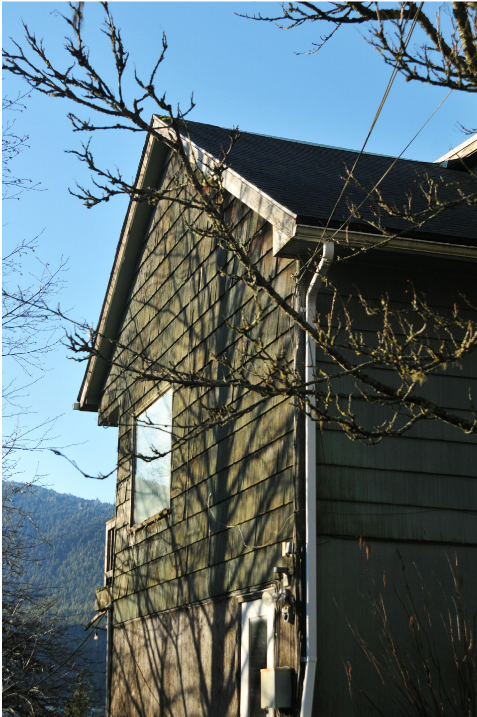
South Facade featuring a contemporary picture window and an entrance to one of the three basement units. Shake-Shingle siding covers the entire residence. Peterson-Kasnick House, 2023
