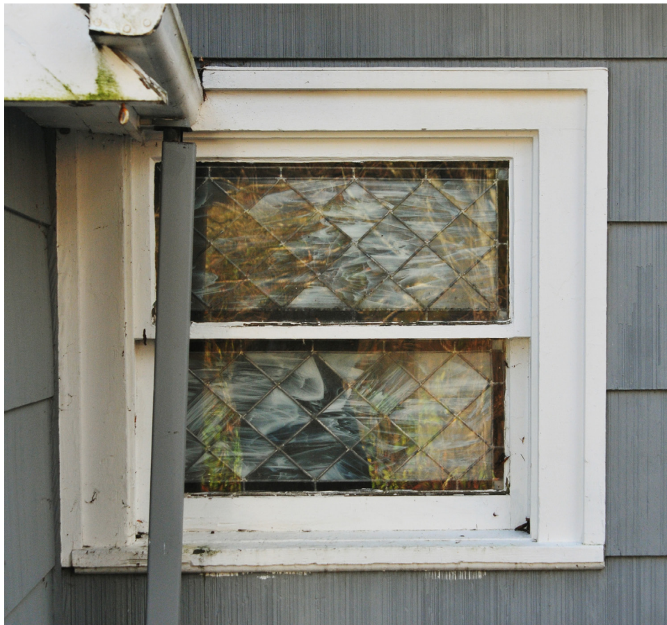
East Facade. Retention of diagonal leaded glass patterned window. Martin-Johnston House, 2023
