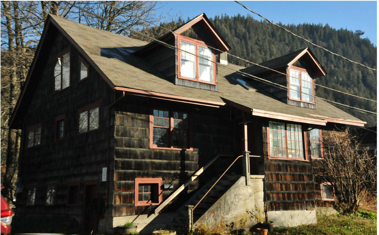
South Facade. Original, double-hung sash windows and original cedar shake siding retained. Wooden gutter has been replicated and replaced in the 1980s. Bayless-Powers House, 2023
