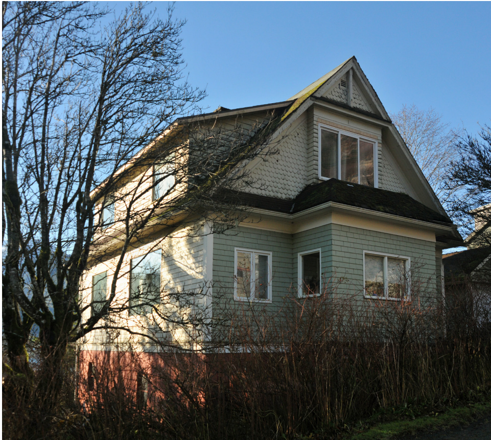
Contemporary additions include the picture windows and dormer on the south facade Bosch-Carrigan House, 2023
