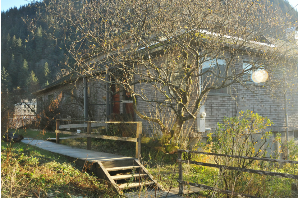
North Facade, main entrance Edward Webster House, 2023
