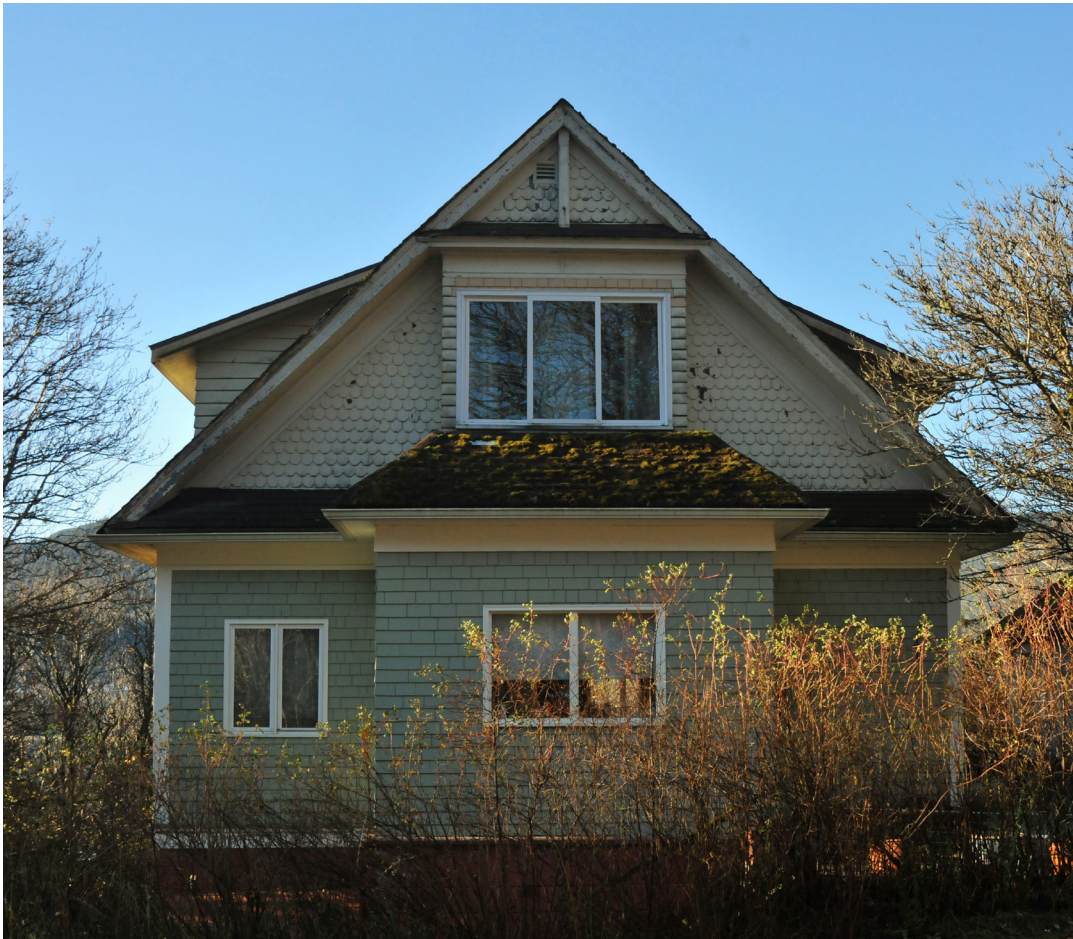
East Facade Bosch-Carrigan House, 2023
