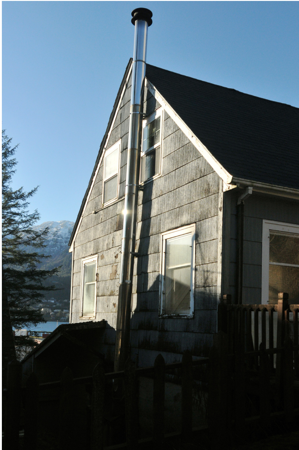
South Facade. A metal chimney has since replaced the original cement block chimney. Martin-Johnston House, 2023
