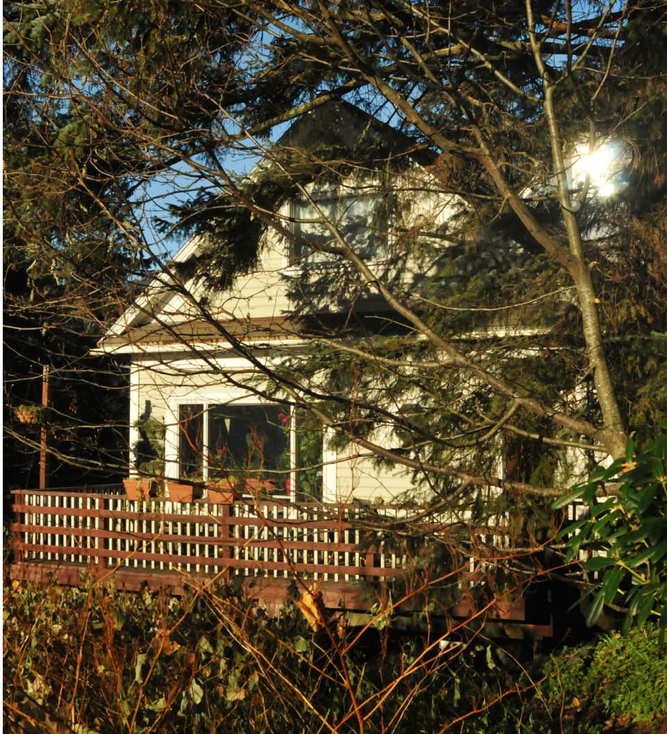
South Facade. Picture windows are placed under the gable and at the main level of the residence. Augustus-Brown House, 2023
