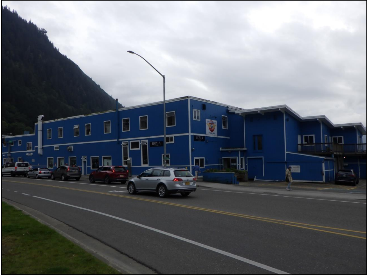
Figure 20. Looking southeast at the Pacific Coastal Steamship Wharf from Egan Ave. (JUN-00120) (NLURA photograph).
