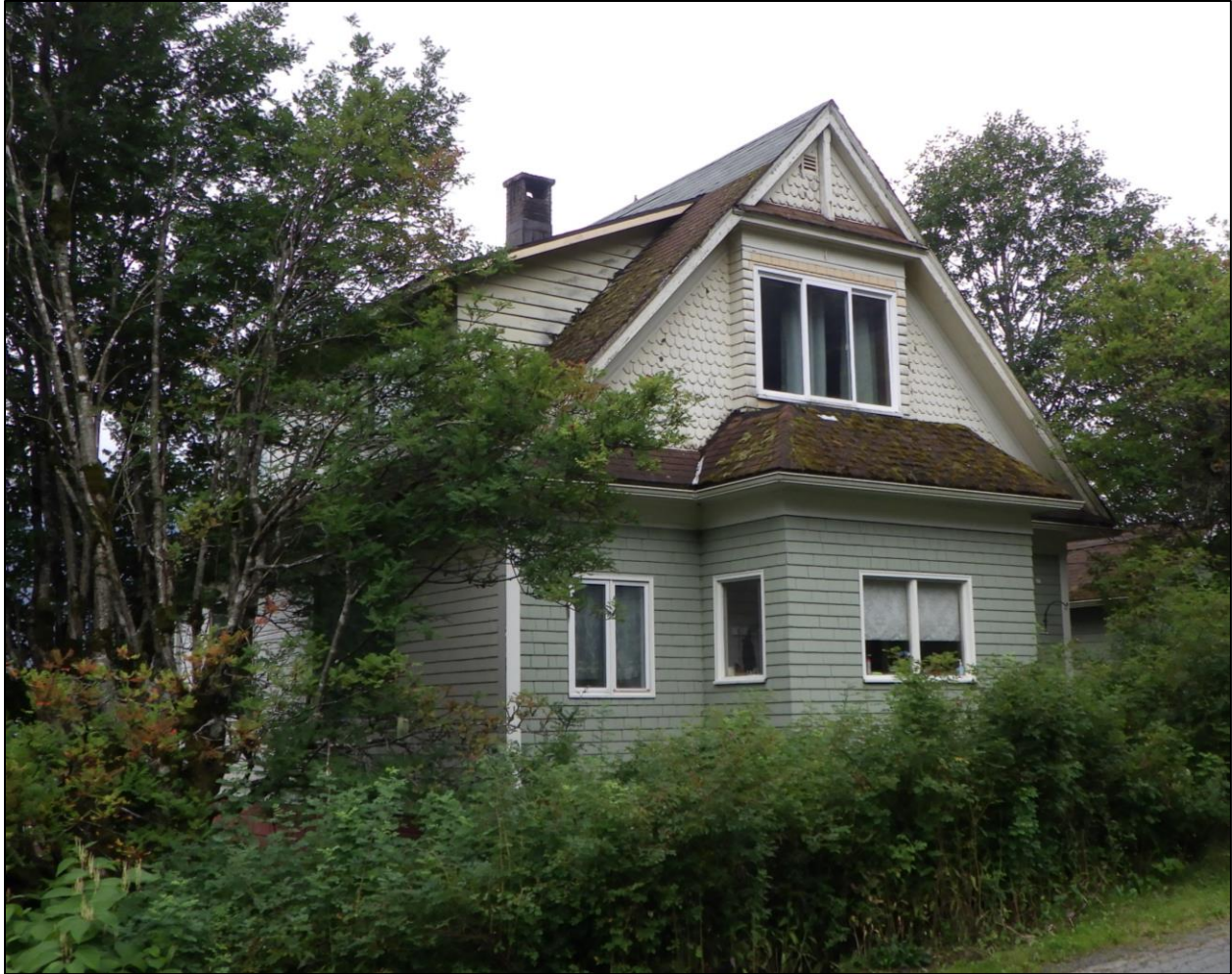
Figure 7. Looking west from Dixon St. at the Bosch/Carrigan House (JUN-00291). Note the Victorian style shingles in the gable end (NLURA photograph).
