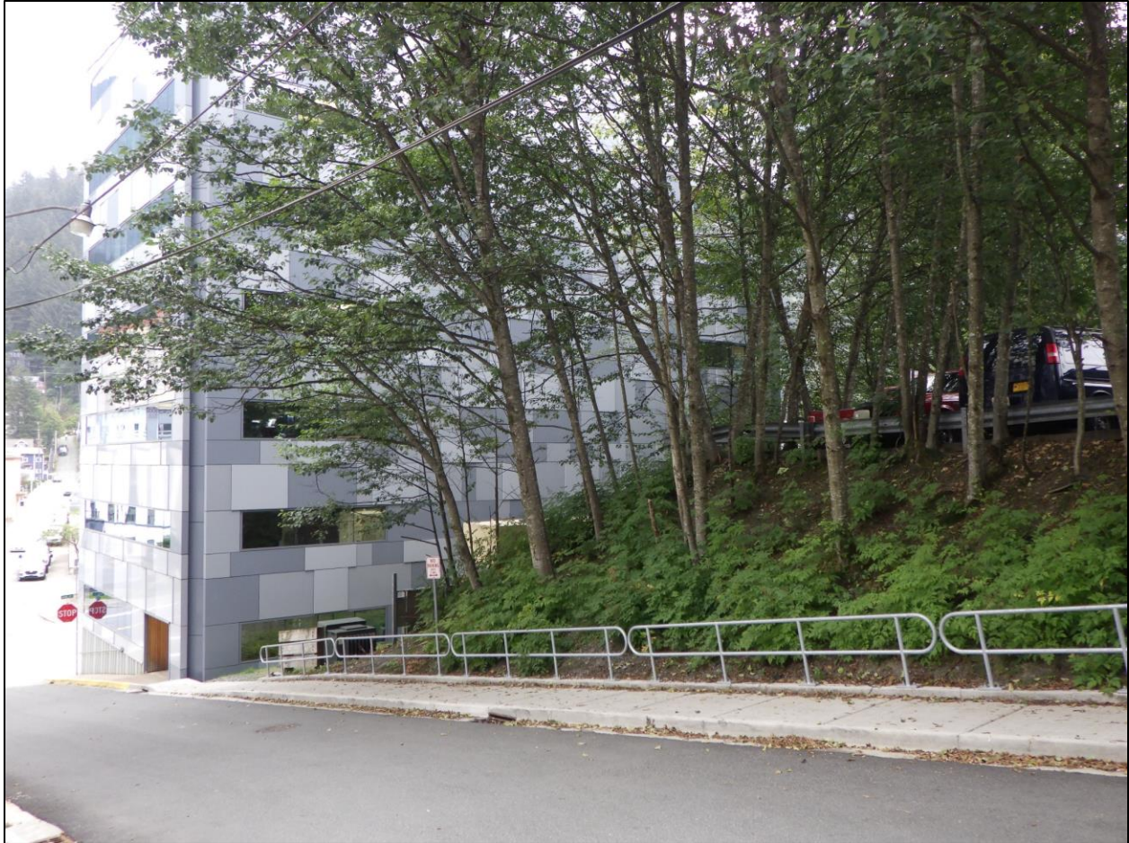
Figure 18. Looking roughly east from West 3rd St. at the former location of the Engstrom Building (JUN-00981) showing the site is demolished (NLURA photograph).
