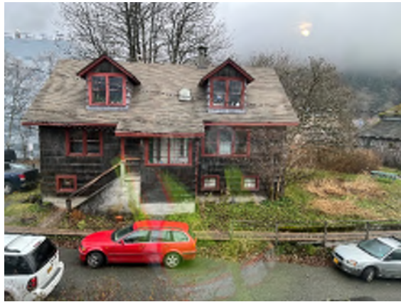
Figure 6-1. West Side of the Building.
