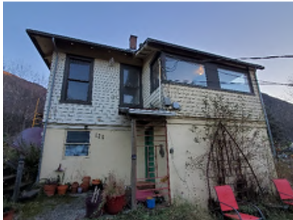
Figure 2-1. West Side of the Building.
