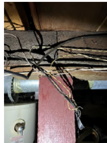
Figure 7-51. The Top of the Column Has a Shim. Even if toe-nails were present, it may not reach the beam its supporting.
