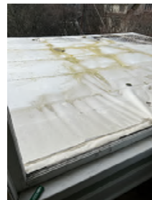
Figure 4-12. Tarp Covering the West Roof.
