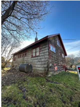
Figure 6-7. East Side of the Building.
