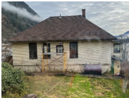
Figure 2-11. North Side of the Building.
