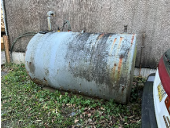
Figure 7-7. A Rusted Tank That Is Not Seismically Secured.
