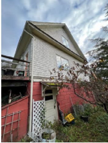
Figure 5-7. Northwest Side of the Building.
