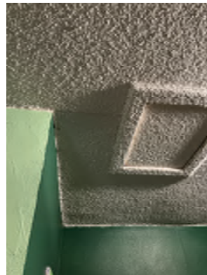
Figure 5-22. Cracked Ceiling Drywall.
