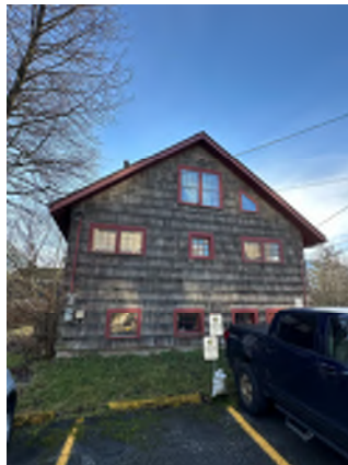
Figure 6-5. North Side of the Building.
