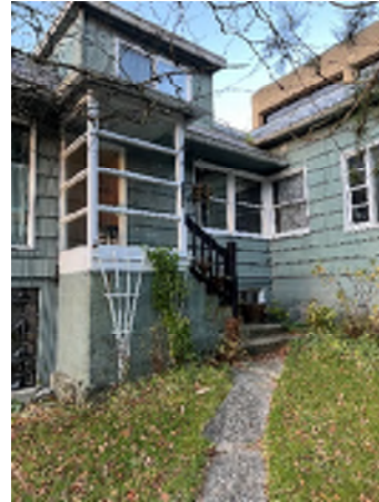
Figure 7-2. There Is Some Deterioration to the Exterior, Including a Cracked Window and Spalled Concrete.
