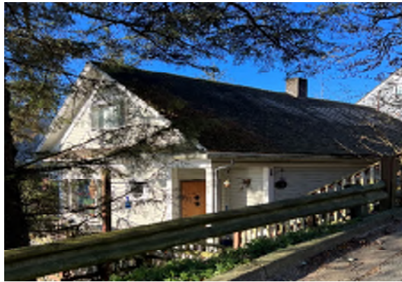
Figure 1-1. South and East Side of the Building.
