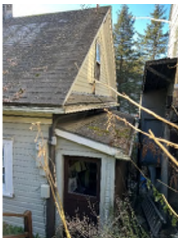
Figure 1-11. North Side of the Building.
