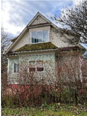
Figure 5-1. East Side of the Building.
