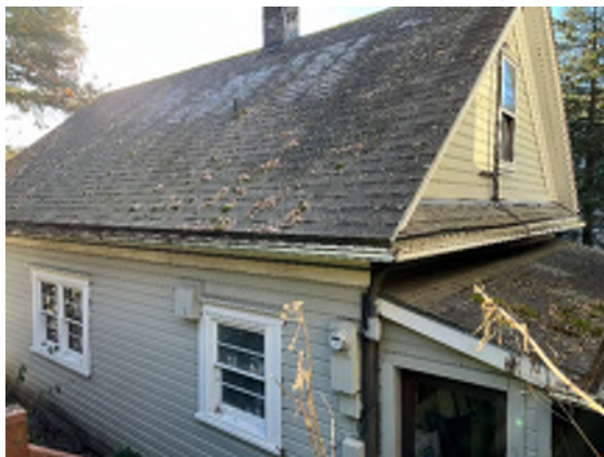
Figure 1-15. East Side of the Building With Wooden Gutters.
