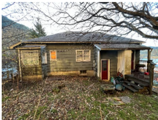
Figure 7-17. North Side of the Building.
