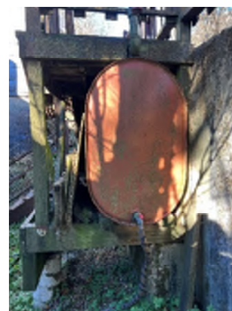
Figure 1-18. The Stair Member Was Cut to Allow for the Vent Pipe at the Top of the Tank.
