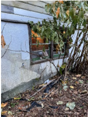
Figure 1-7. Replaced and Repainted Pieces of Siding.
