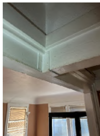
Figure 3-30. A Beam Hanger Observed at the Framing Near the Stair Opening.
