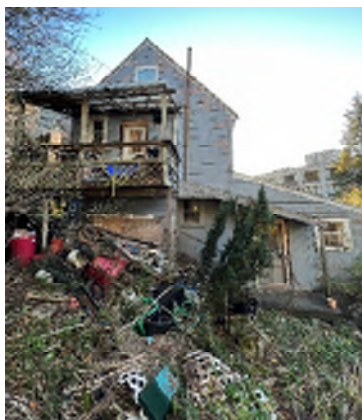
Figure 3-5. North Side of the Building.
