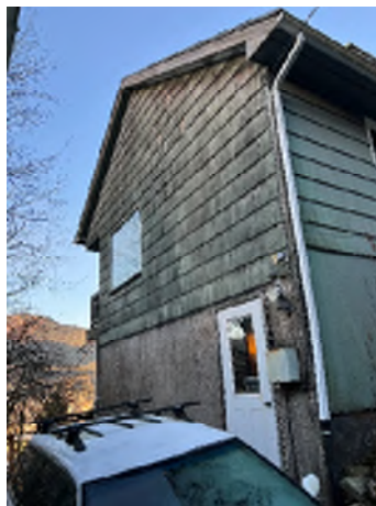
Figure 7-5. South Side of the Building.
