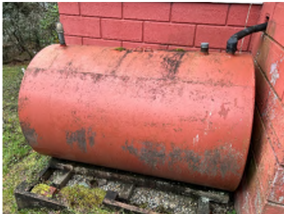
Figure 5-3. Cracking in the Concrete Wall. The tank is not seismically anchored and the framing is rotten.
