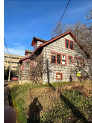
Figure 6-12. South Side of the Building.
