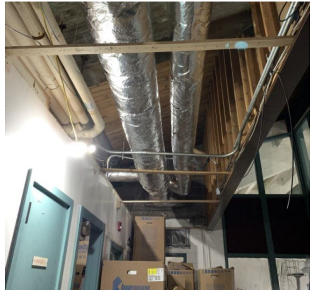
New HVAC ducting installed in lobby ceiling.
