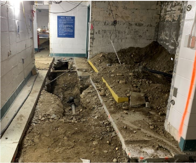
(Above) Finished replacing old plumbing and beginning the process of filling in around new pipes in Woman's Locker Room.
