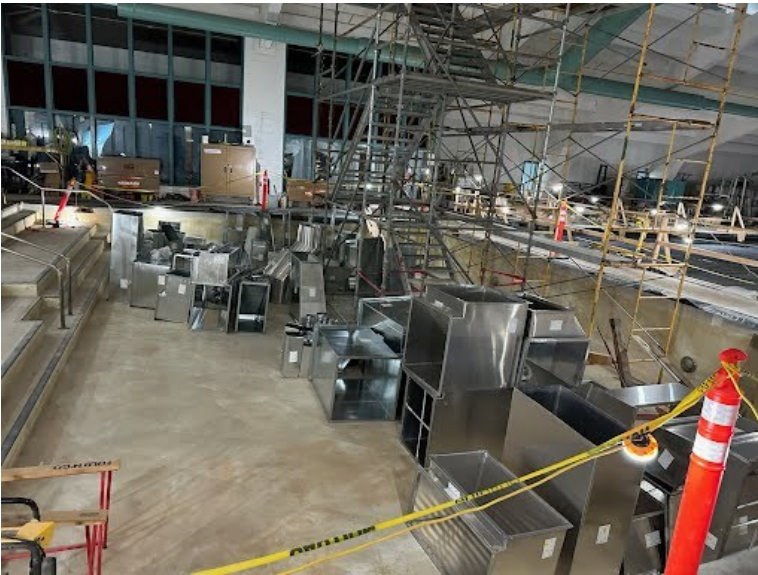
New HVAC ducting staged and ready to install.
