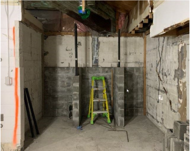
(Below) ADA accessible showers in Woman's Locker Room being constructed. Increased from two to three showers.
