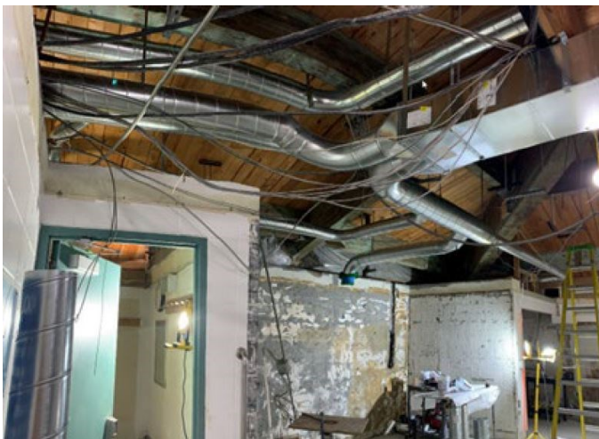
New HVAC ducting installed in Woman's Locker Room.
