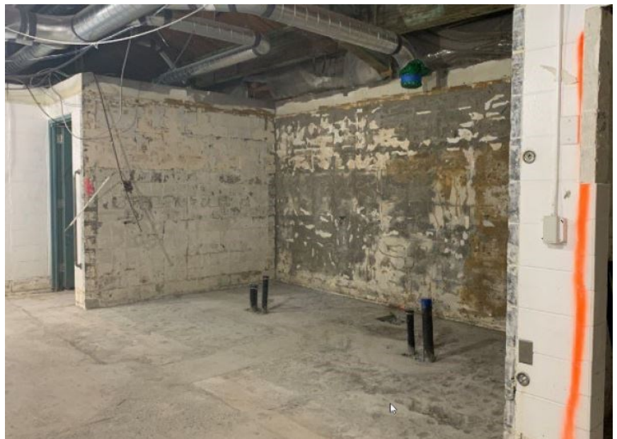
(Right) New concrete poured and sloped in preparation for new tile floor in Woman's shower area.
