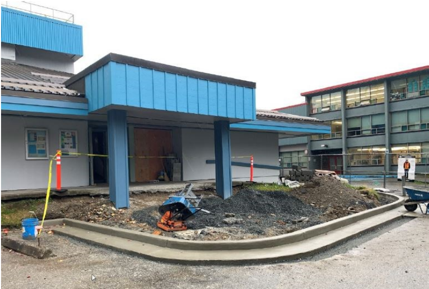
(Right) New curb for front entry pad poured
