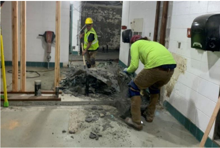
(Above) Demoeing the floor in toilet area in Locker Rooms to prepare for new plumbing and fixtures.
