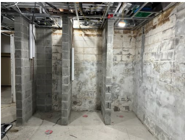
ADA accessible showers in Men's Locker Room ready for tiling and fixtures.
