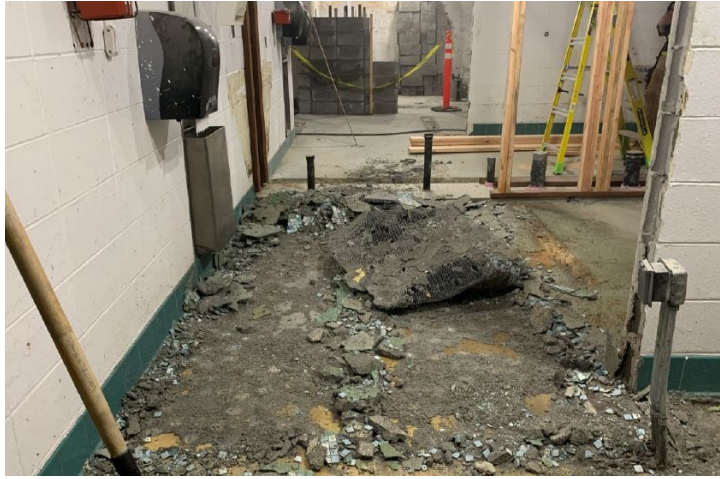
(Above) Floor demoed and new pluming run Woman’s locker room toilet area.
