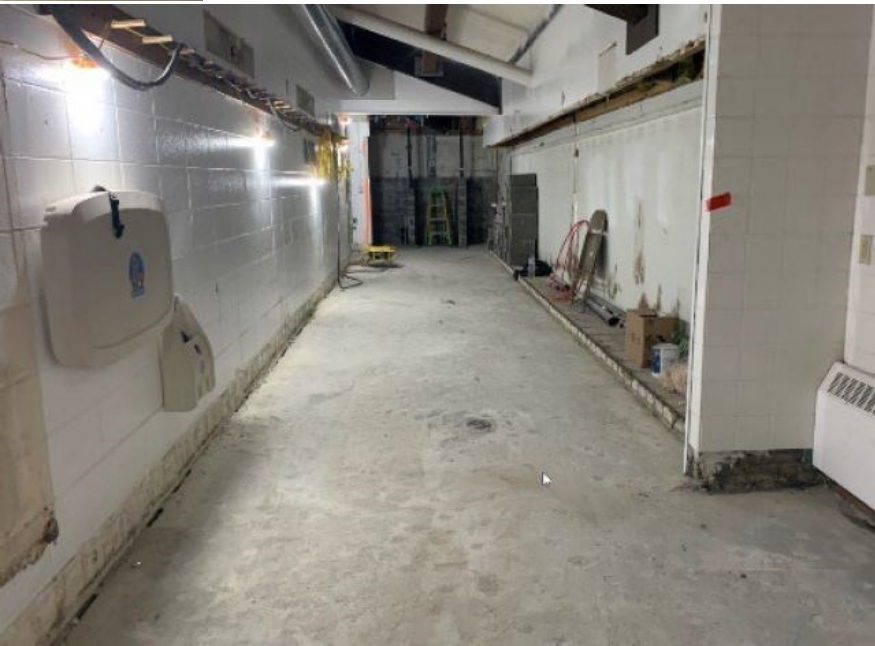
(Left) Preparing the floor in Woman's locker room. Removed old epoxy and tile flooring and set new grade with fresh dry pack mortar.
