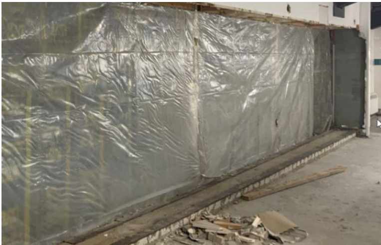
(Left) Preparing the floor in Woman's locker room. Removed old epoxy and tile flooring and set new grade with fresh dry pack mortar.
