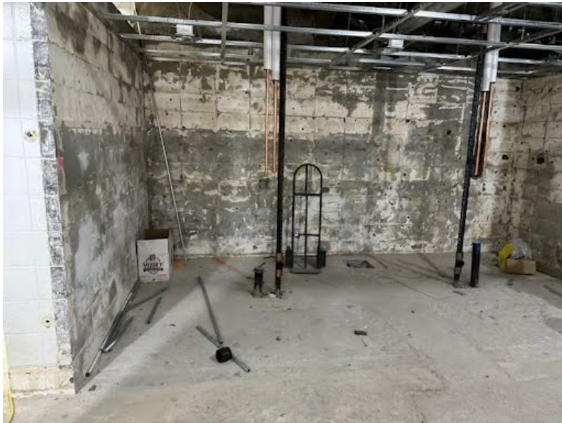
(Above) Finished replacing old plumbing and beginning the process of filling in around new pipes in Woman's Locker Room.
