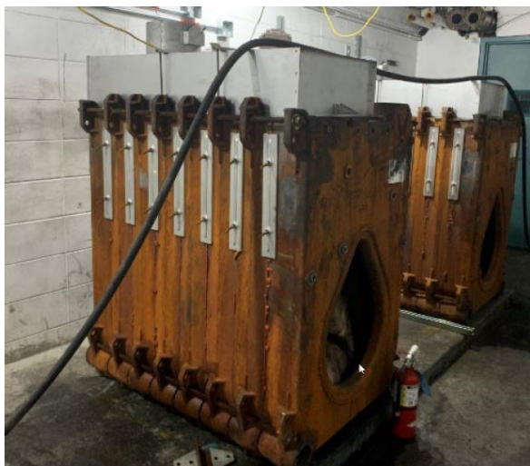
(Above) New Boiler units set into place and ready for their outer casing.
