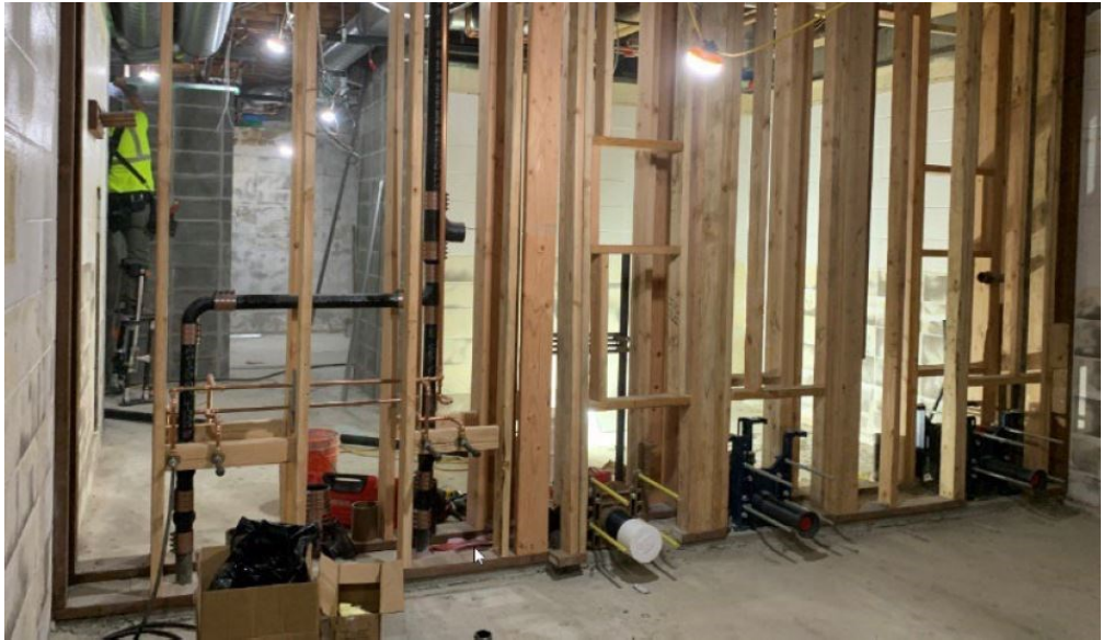
(Right) Opposite view of new plumbing wall installed between Woman’s and Men’s locker room toilet areas.
