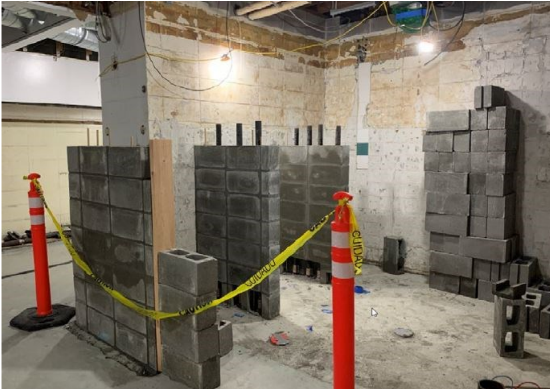
(Above) Constructing ADA accessible showers in Men's Locker Room.
