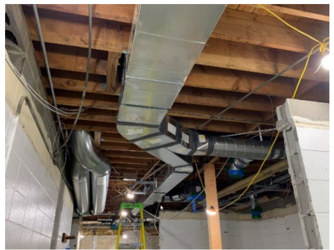
New HVAC ducting installed in Men's Woman's Locker
