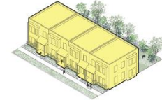
Two-story attached houses
