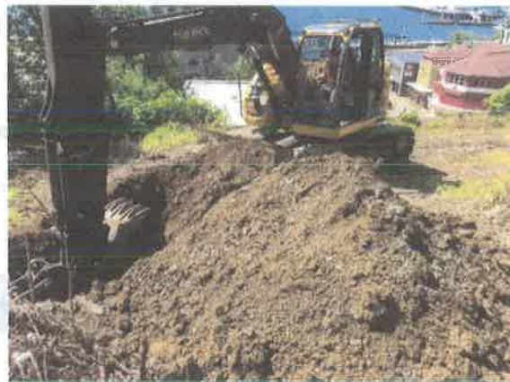
Figure 3: Excavator and in-situ silty sand with gravel
