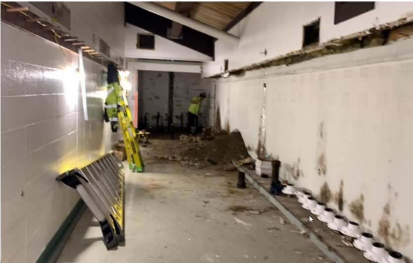
Demo work in woman's locker room. Lockers removed and [moldy] sheet rock (to be replaced) exposed.
