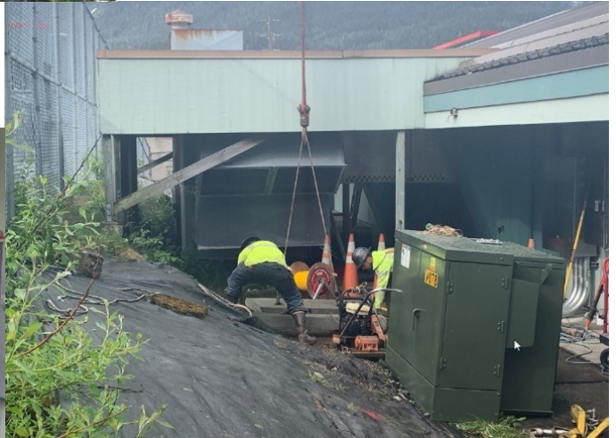
(Left) ALCAN electricians installing the new transformer building hook ups.
