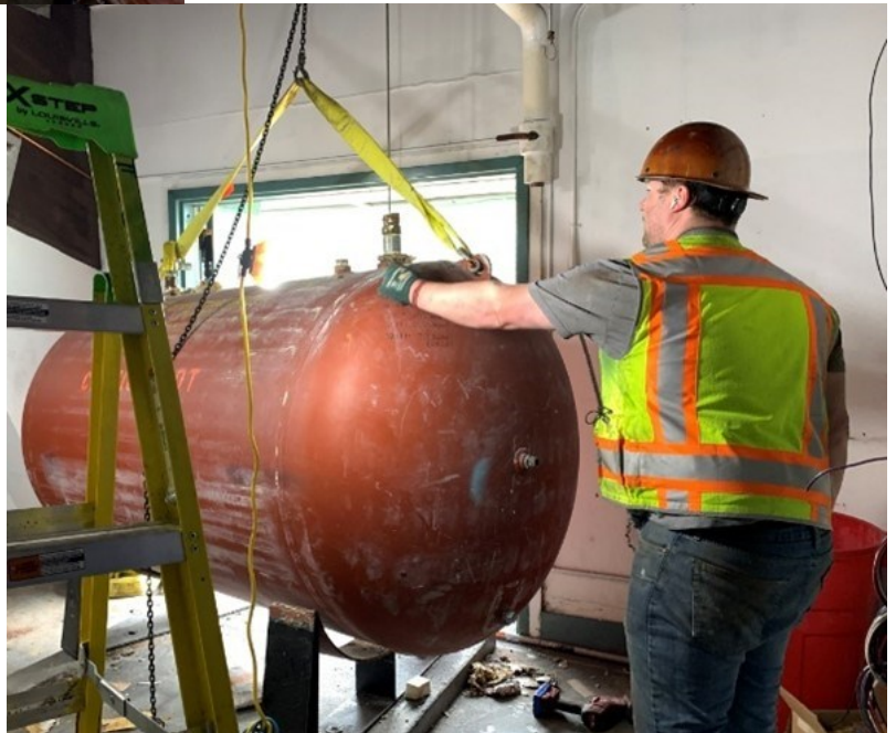
(Right) Removing old hot water storage tank.
