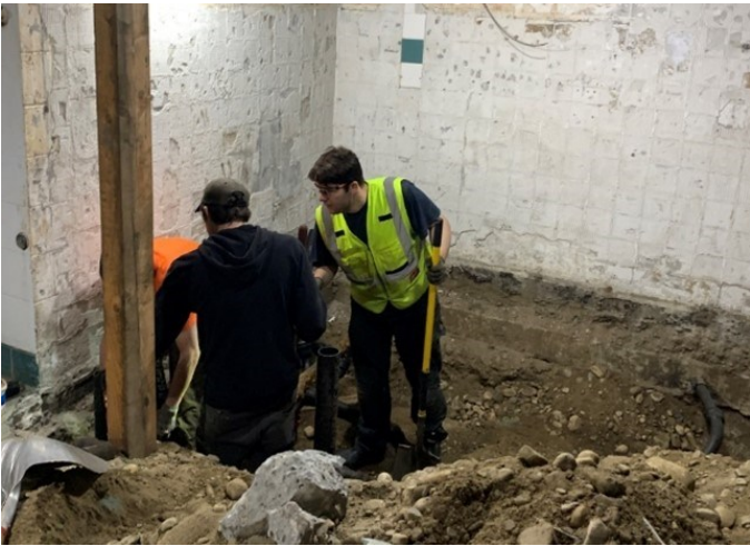
Demo work in men's shower area. Temporary support beam for installation of new ceiling joist.
