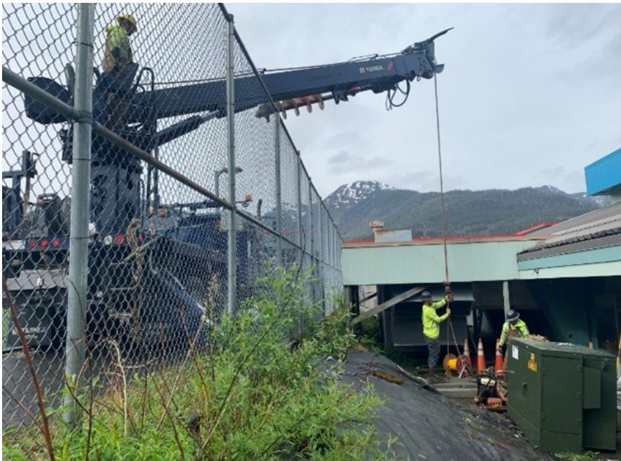
(Left & below) AEL&P boom truck and AL-CAN electricians preparing to install new transporter.
