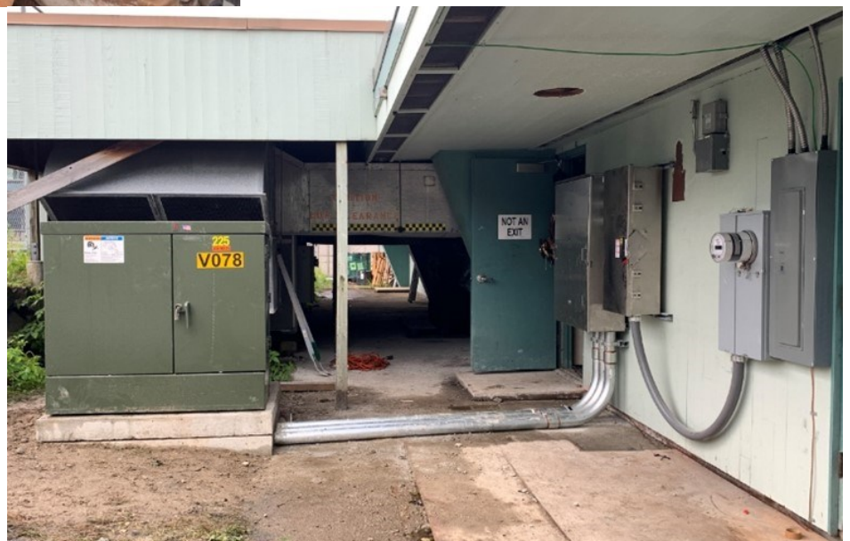
New transformer installed and hook up.
