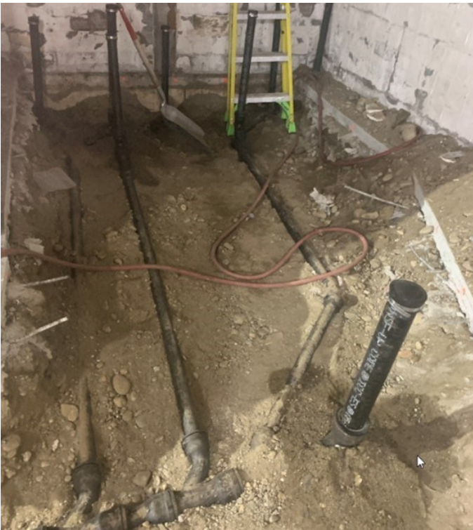
New plumbing and drains for men's locker room shower area.
