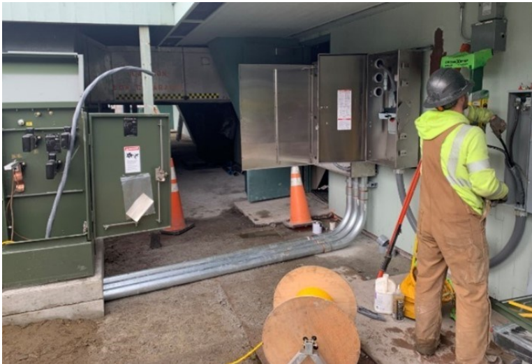
(Left) ALCAN electricians installing the new transformer building hook ups.
