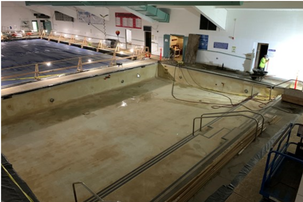
(Above left and right) Demo to pool deck outside of sauna to prepare for the replacement of old and damaged drainage pipes.
