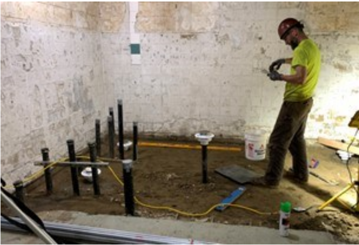
New plumbing and drains for ADA accessibility shower stalls in men's locker room.
