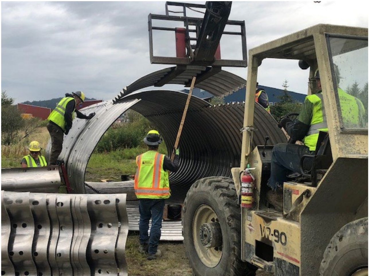
SECON assembling the new culvert sections on site.
