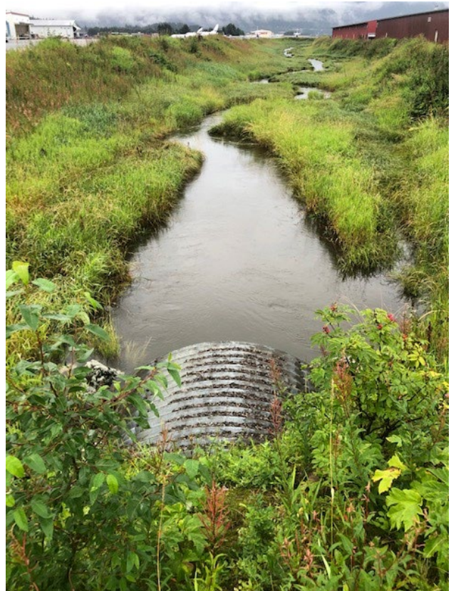
Photo 02: Culvert outlet in Jordan Creek.
