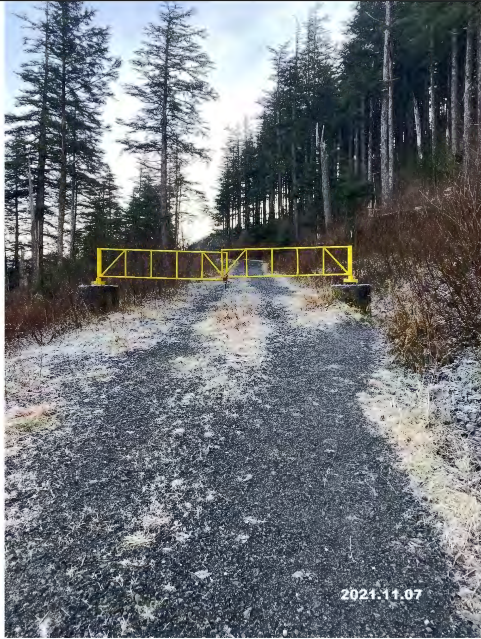
Gate at Access Road from John Street
