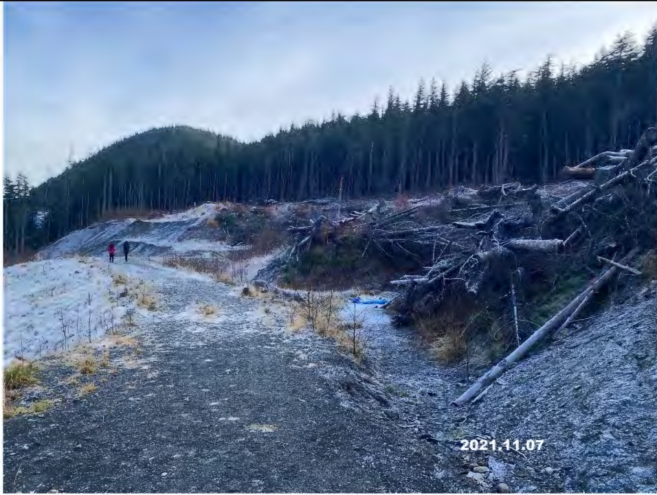
Partially Cleared Portion of Parcel
