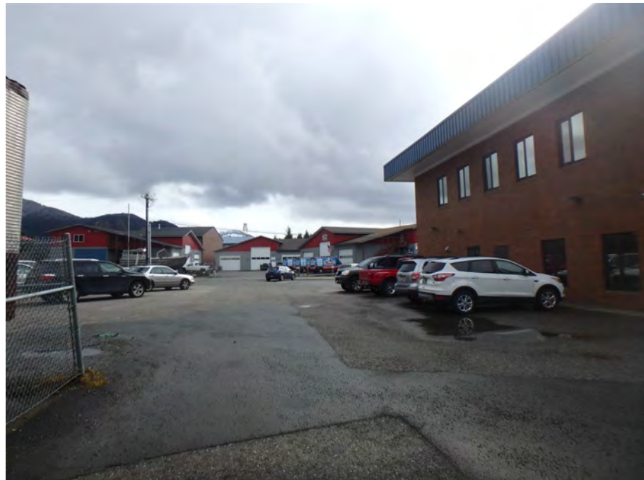
Looking north along rear of subject from southwest corner
