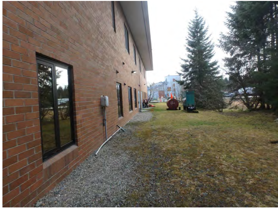
South side of subject with generator and fuel tank
