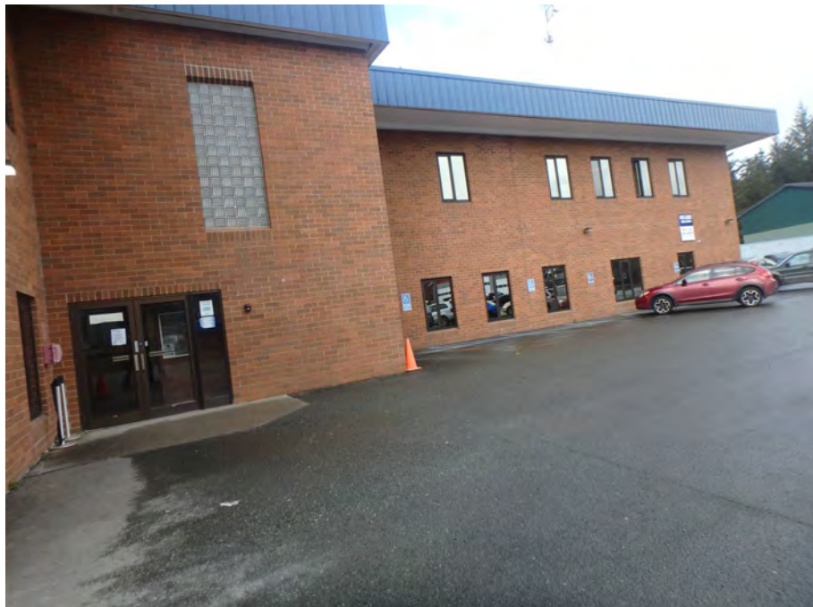
Looking west at subject front lobby door
