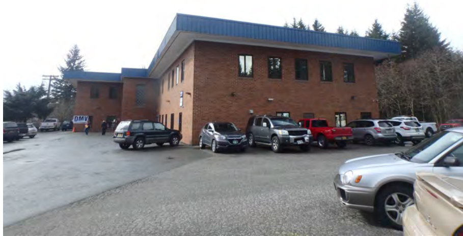
Looking southwest at subject
