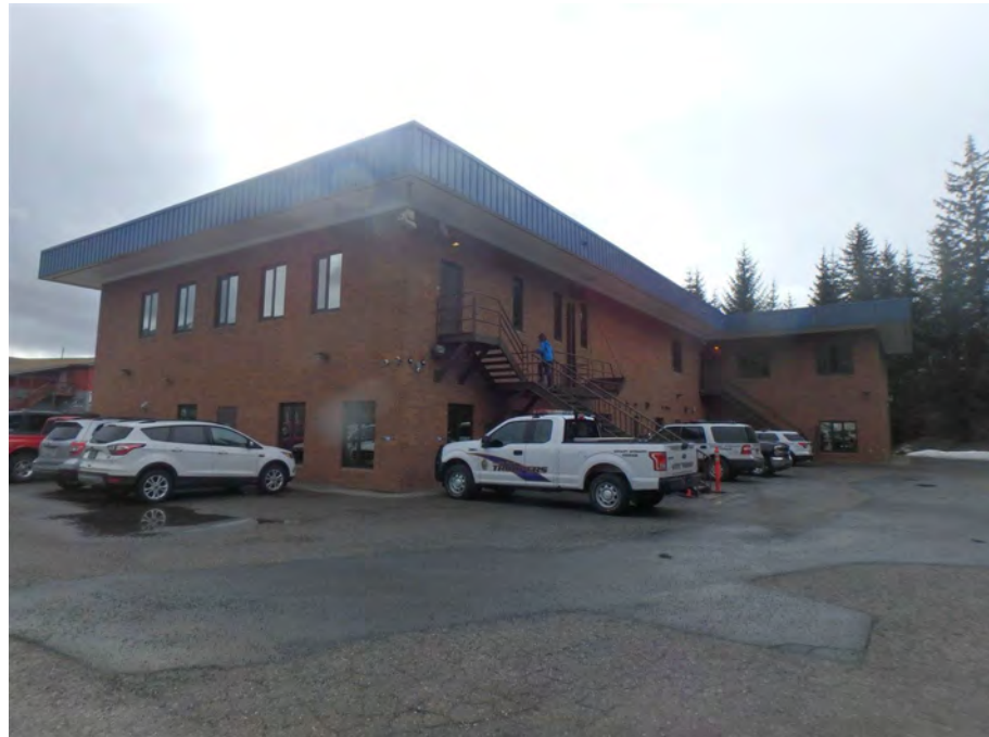
Looking south at rear of subject
