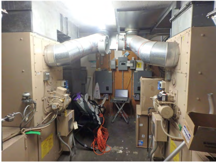
2 nd floor mechanical room
