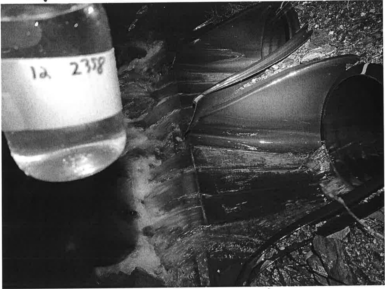
OUTFALL 12: TWY D-E INFIELD DRAINAGE
