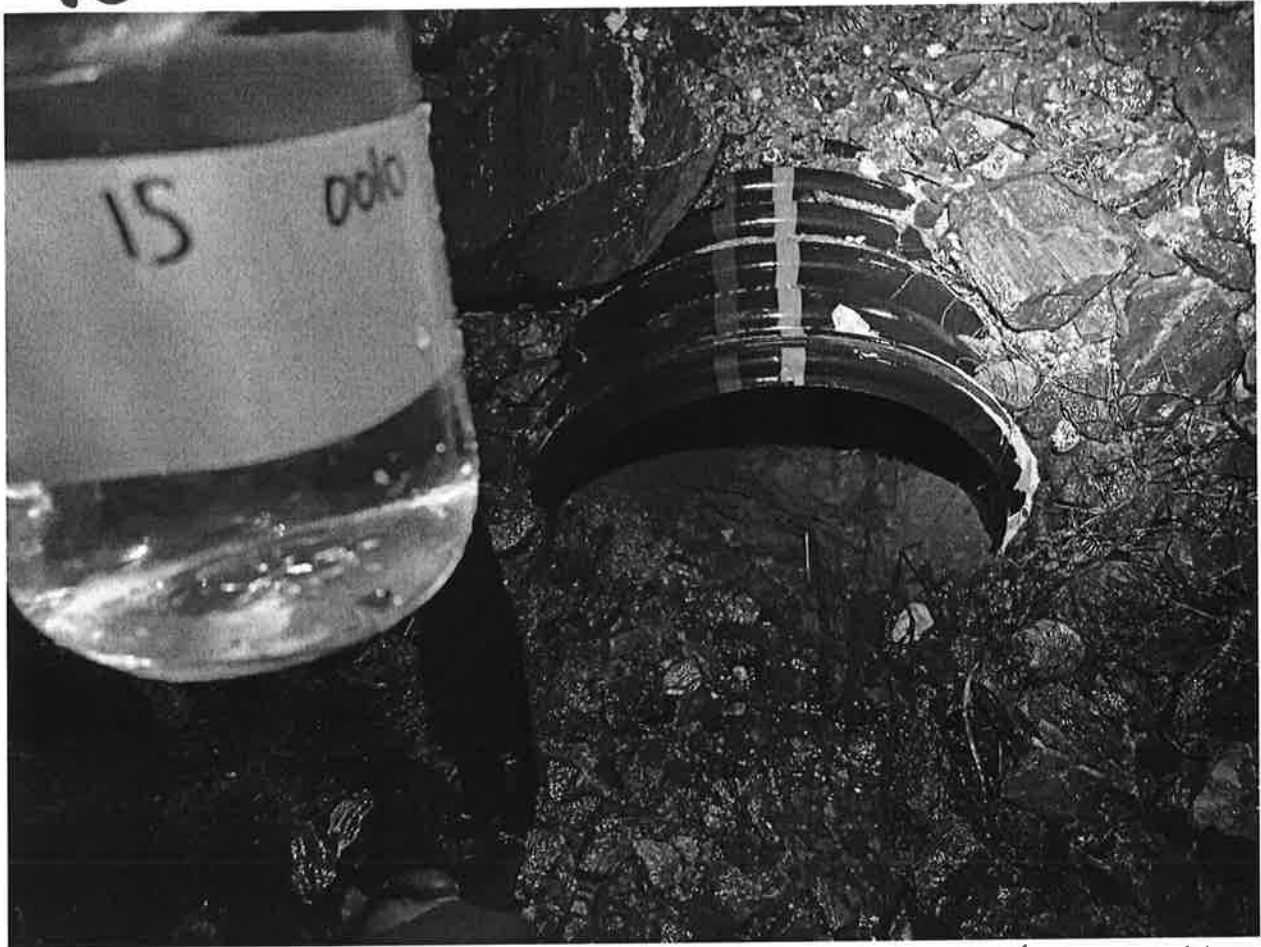
OUTFALL 15: Pond Parking Area Outlet
