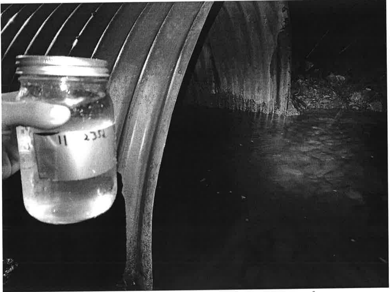
OUT FALL 11: Jordan CRK Culvert outlet
