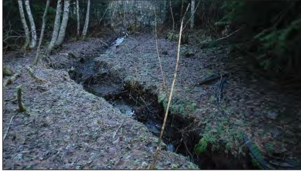
Figure 2.—Channel at toe of fill.
