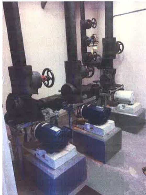
Mountainside Estates Pump Station
