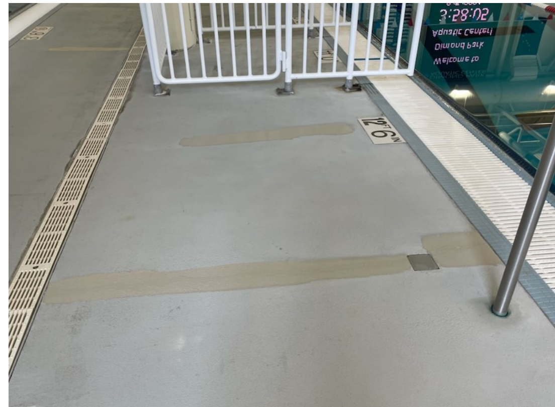
PHOTO AFTER REPAIRS.
