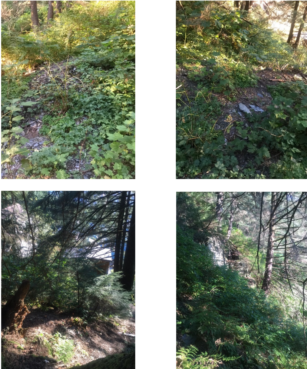
Figure 9: Photos at the top show active debris slide paths above Nelson Street; photos at the bottom show rock bluffs and broken or damaged trees above Nelson Street.
