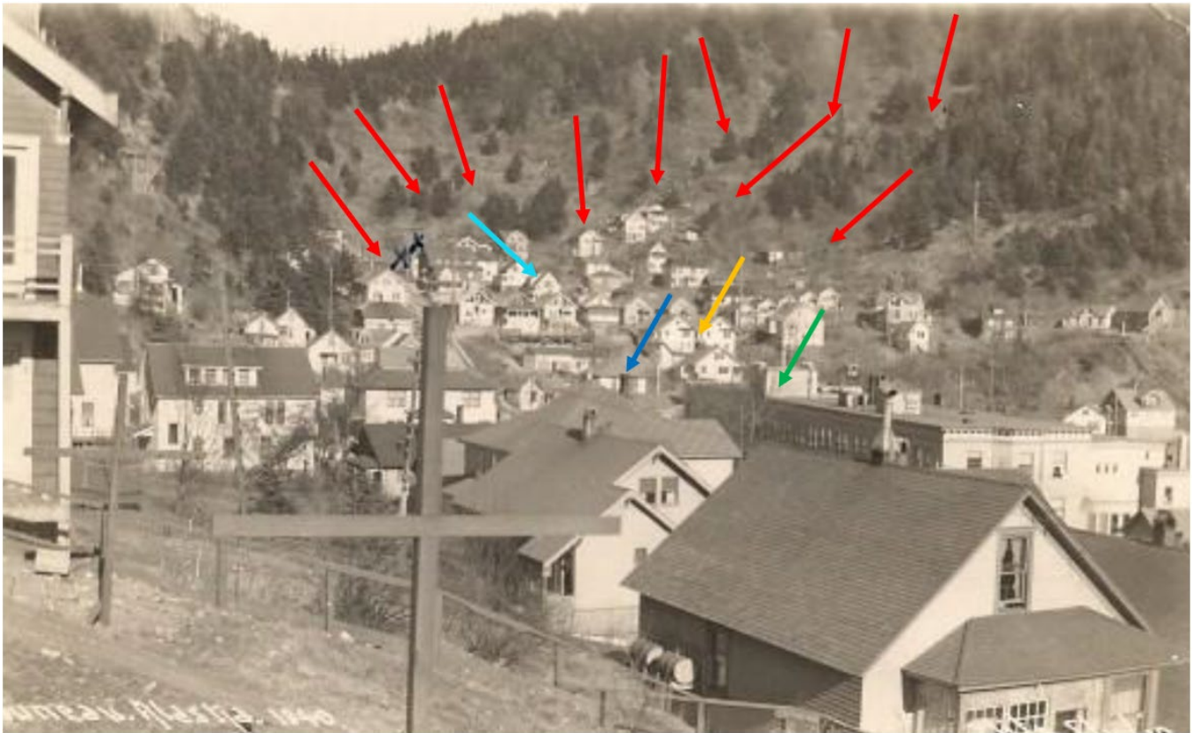
Figure 10: Looking east-northeast, this view of Starr Hill in 1940 is from a little further southwest of the view in Figure 9, and somewhat foreshortened. After more than 40 years of tree growth after clearcutting, the swales and gullies where no coniferous trees grow are especially clear in this photo. Selected swales and gullies are shown with red arrows; several other swales and gullies are also visible between the red arrows.
