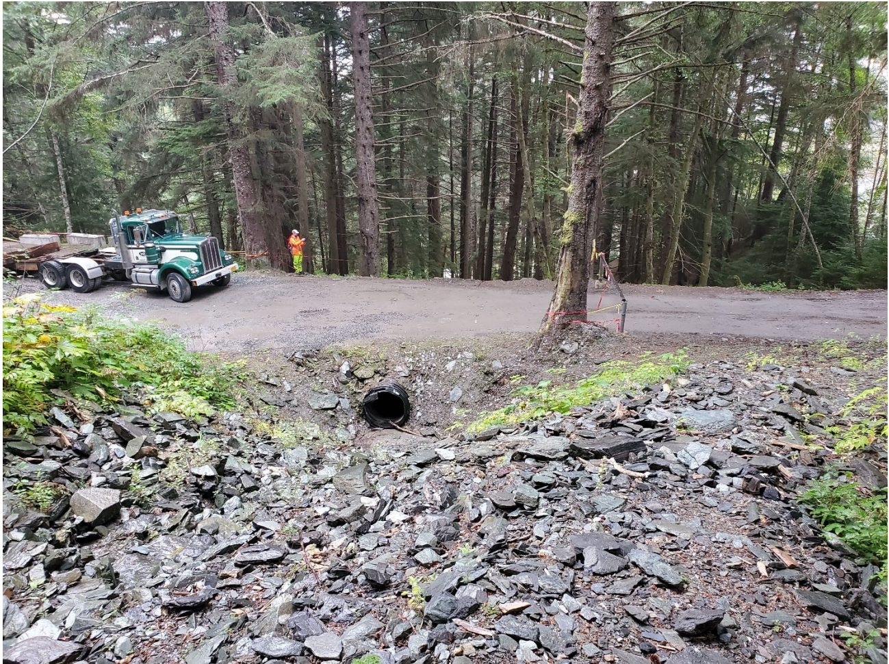
Figure 4: Looking down towards the Gold Creek Flume Trail from the Bathe Creek debris flow gully. Note the large amount of debris in and alongside the gully, as well as the scarring on the tree beside the road that extends to at least 6 feet above ground surface. This gully is very active, and the debris that is deposited at the road crossing is regularly cleaned up. This road crossing has the potential to divert debris flows into the residential community downslope and to the west, especially if more than one surge of debris occurs before the debris can be cleaned.
