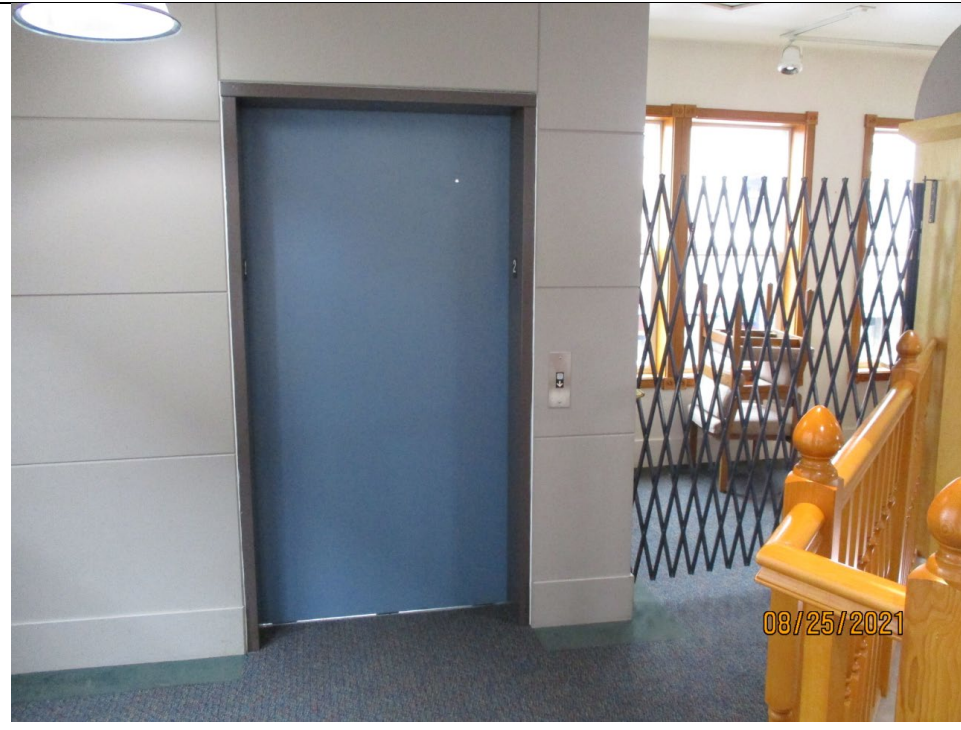
Elevator on 2 nd floor
