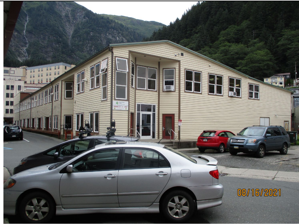
Building and parking as seen from Shattuck Way
