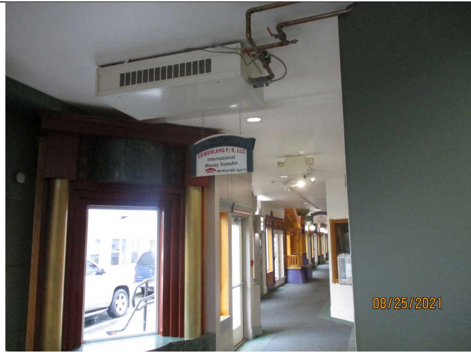
1 st floor hall way along Shattuck Way
