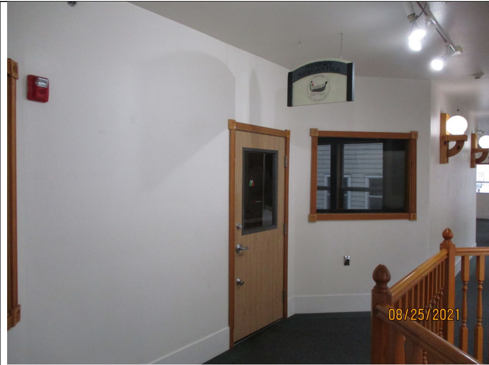
Office space on 2 nd story
