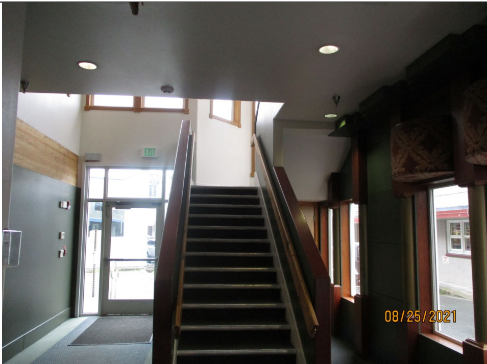
Rear stairway to 2 nd floor
