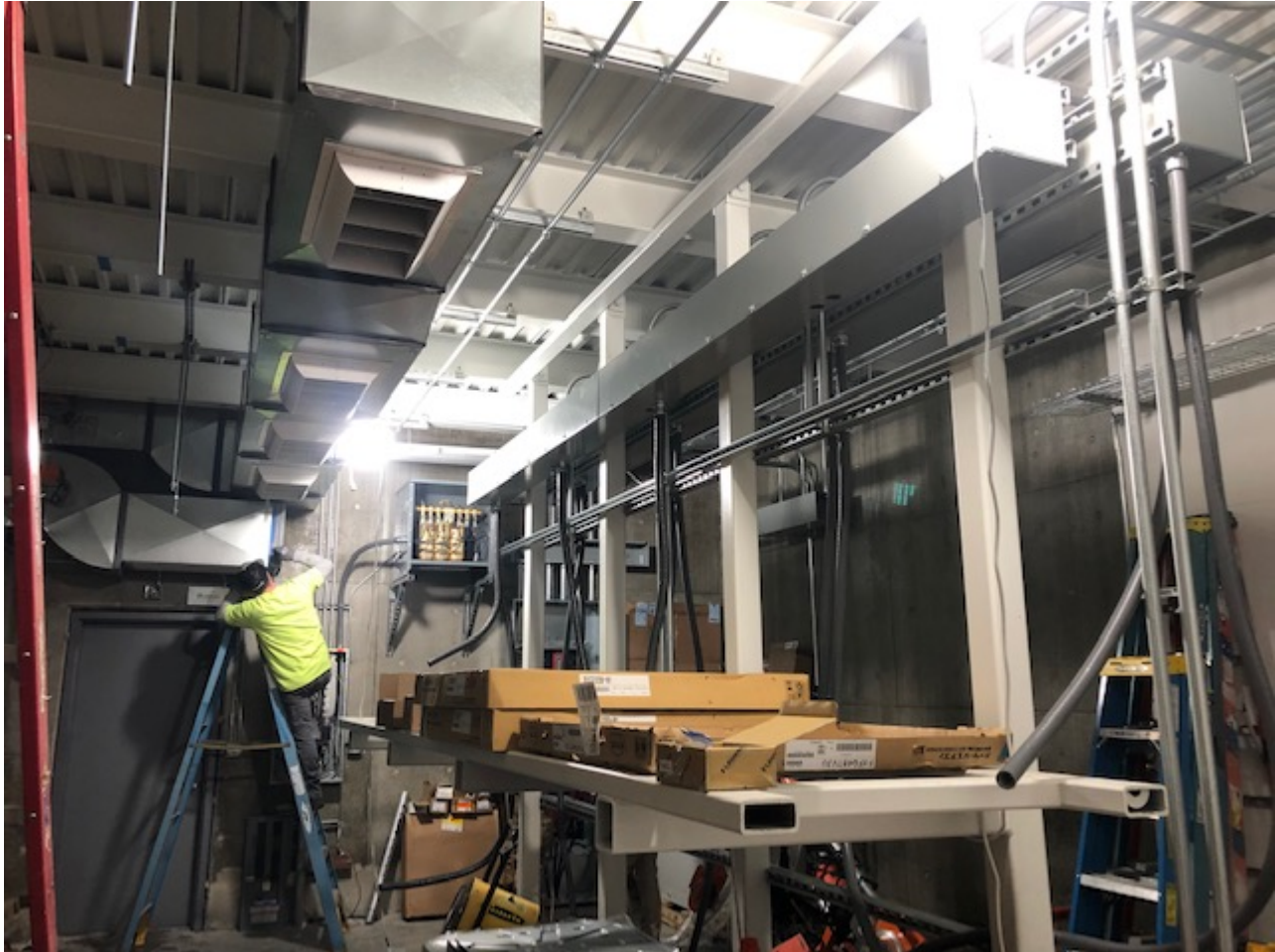
Photo 02: Return air ductwork being installed in the northwest corner of the new ALRV. The new regulator support rack is shown in the center of the photo.
