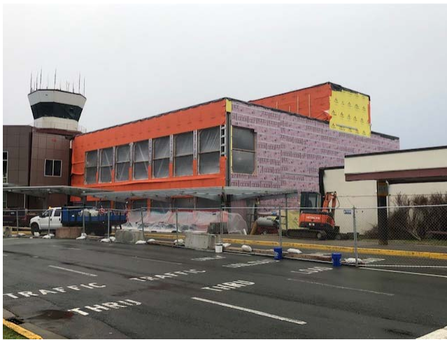
Photo 01: Landside of the terminal.
