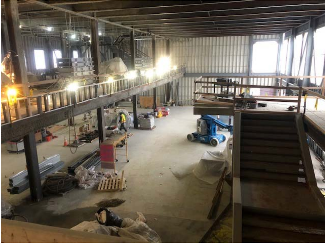
Photo 03: Second floor balcony, interior stair and 135 departure / waiting area.
