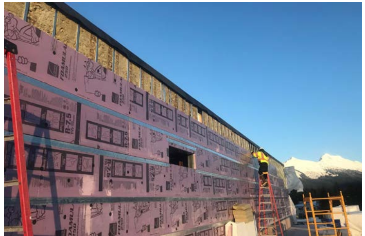
Installing insulation and z-girts on the penthouse exterior wall.
