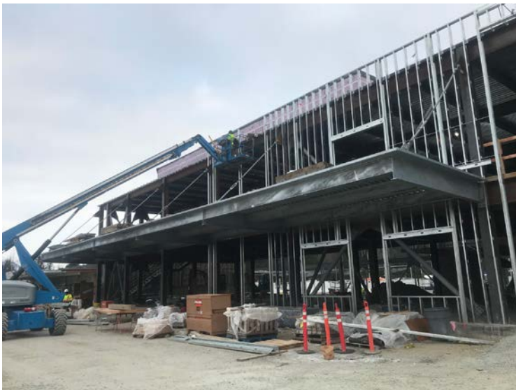
Exterior framing of the west (air side) elevation.
