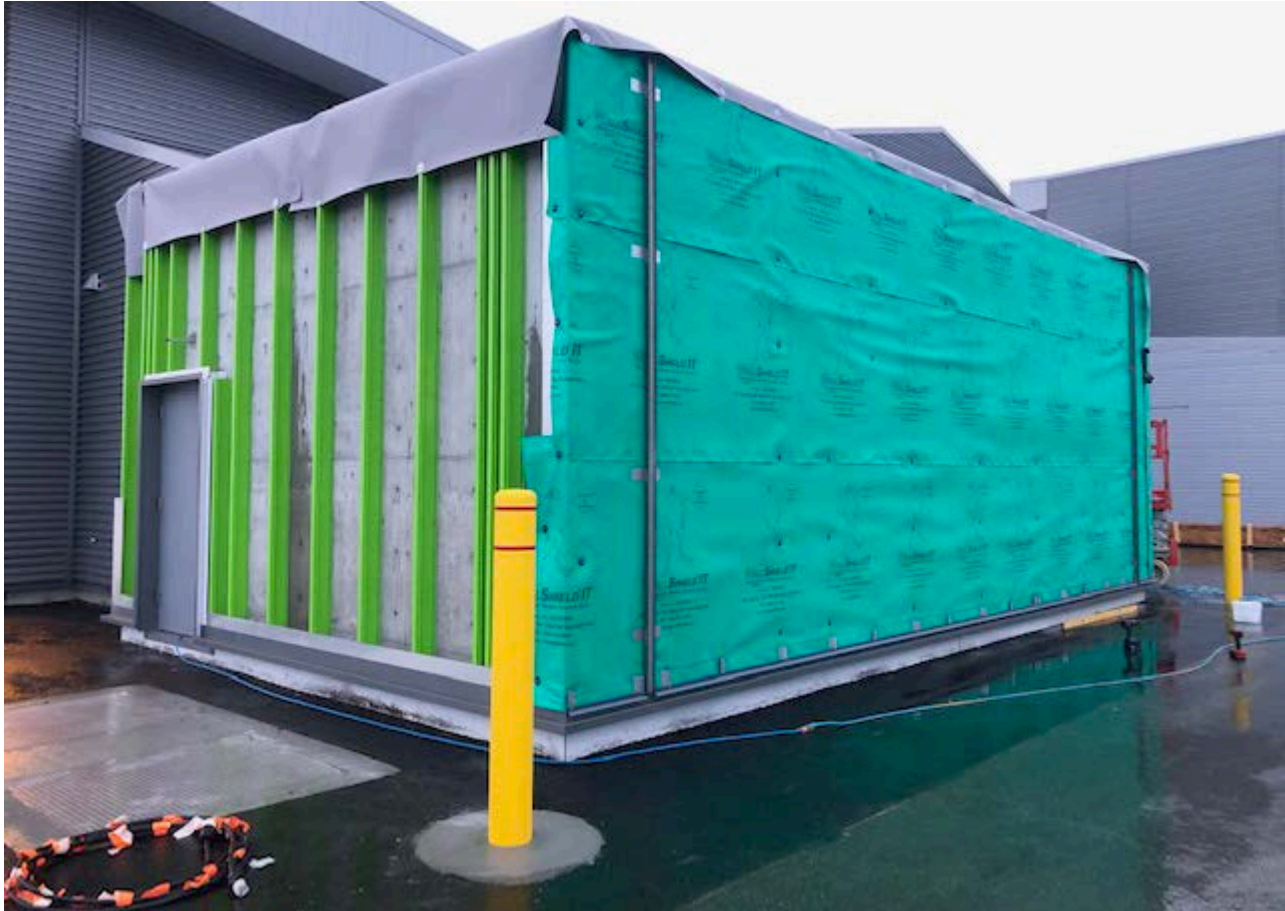
Figure 1-1: Exterior metal siding work underway on the new ALRV addition to the SREB.
