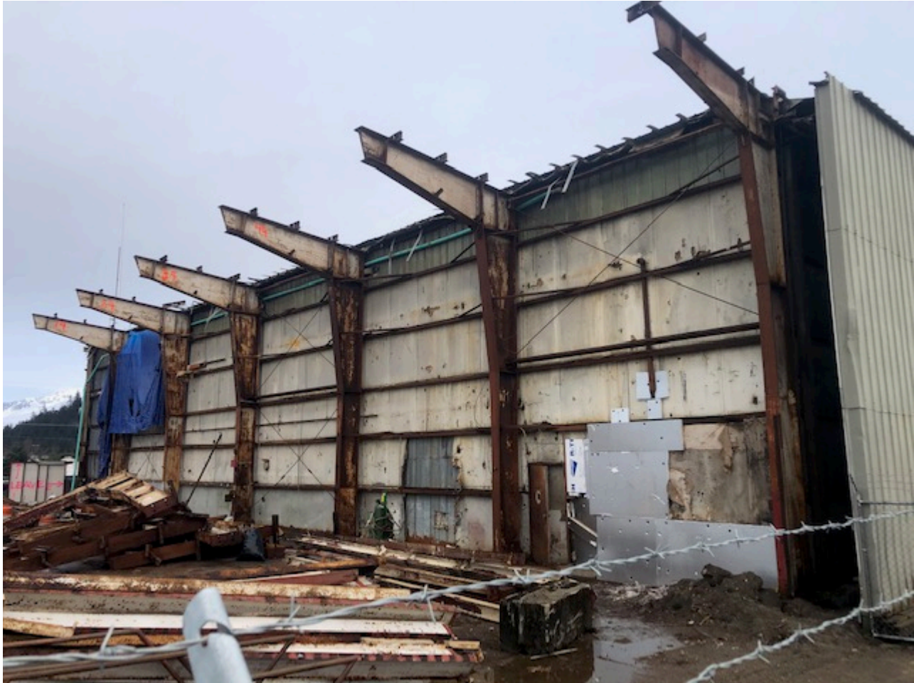
Figure 2-1: Primary steel columns remain in place along the length of the shared wall assembly.
