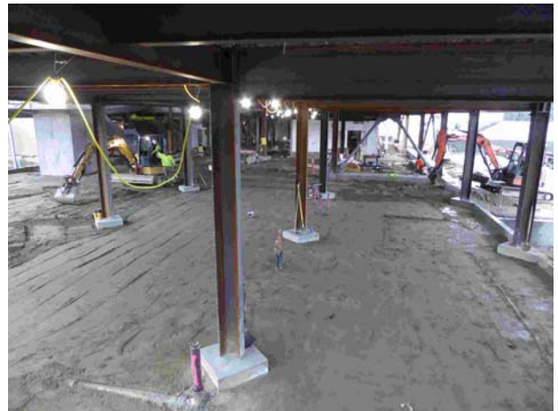
Looking south through first floor regional air carrier spaces.
