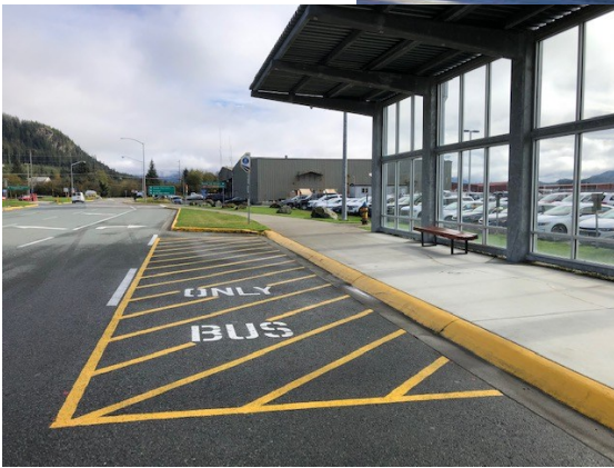
New Capital Transit stop at east end of bus canopy.
