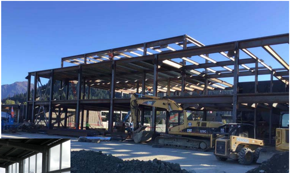
Structural steel frame, looking northeast from airfield side.
