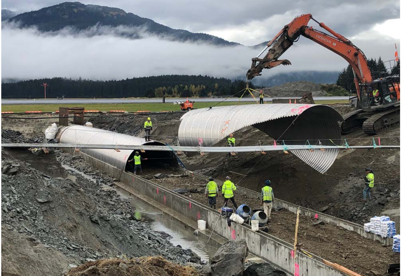
Figure 1-1: SECON crew setting the third half-arch culvert section on top of the pre-cast concrete footings.
