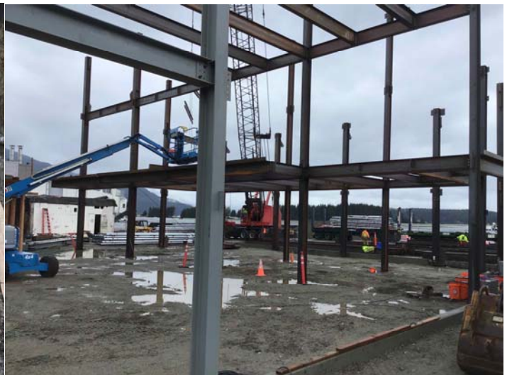
Start of steel erection.
