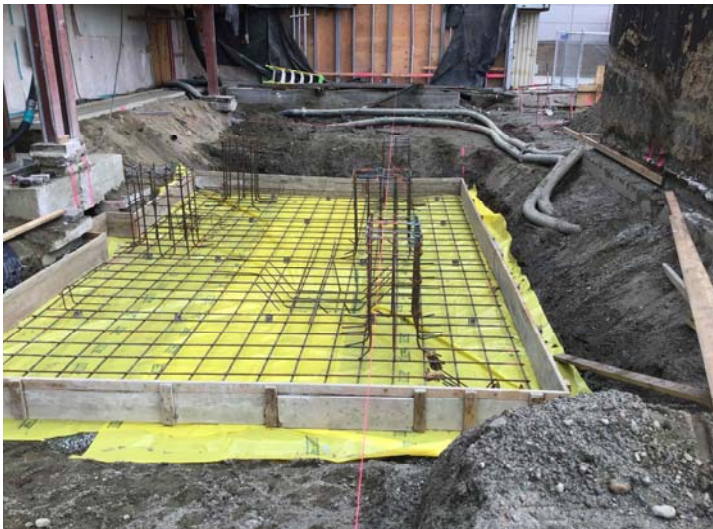
Concrete foundation work.
