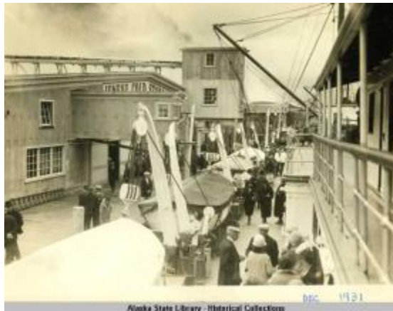
Juneau Cold Storage – December 1931
