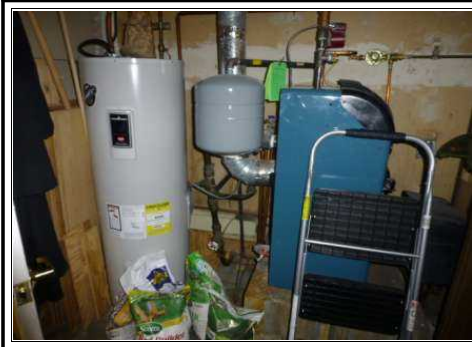
Water Heater and Boiler
