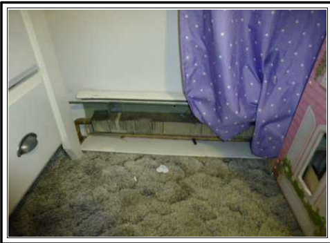
Baseboard Missing Cover
