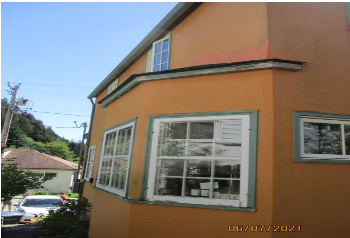
NE Side with Old Windows on 1 st Floor:
