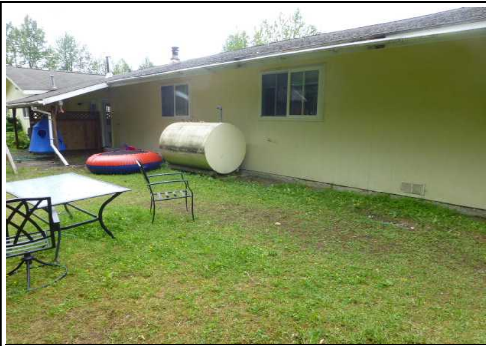
REAR OF SUBJECT PROPERTY
