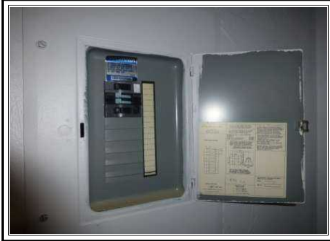
Electrical Panel - Sylvania
