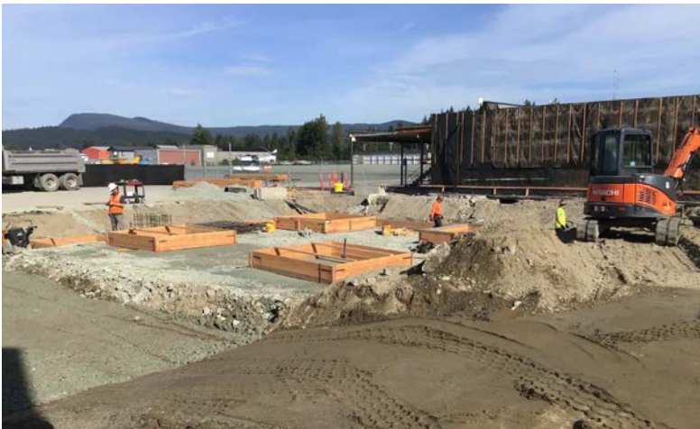
From airside, looking northeasterly into work area.
