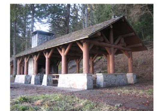
STONE AND TIMBER PICNIC SHELTER
