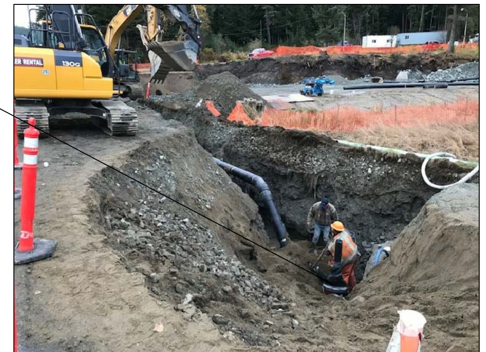
12" MJ GV AND HDPE INSTALL OCTOBER 2018
