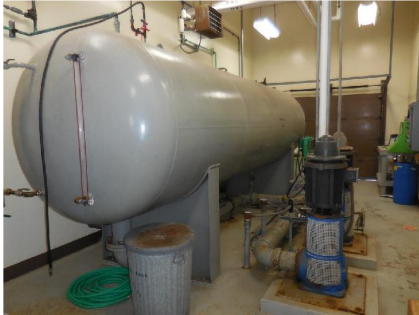
Figure 11. NPW Tank and Pump System
