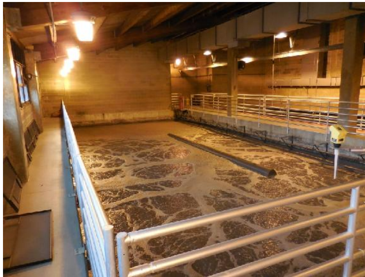
Figure 8. SBR in the Aeration (React) Cycle
