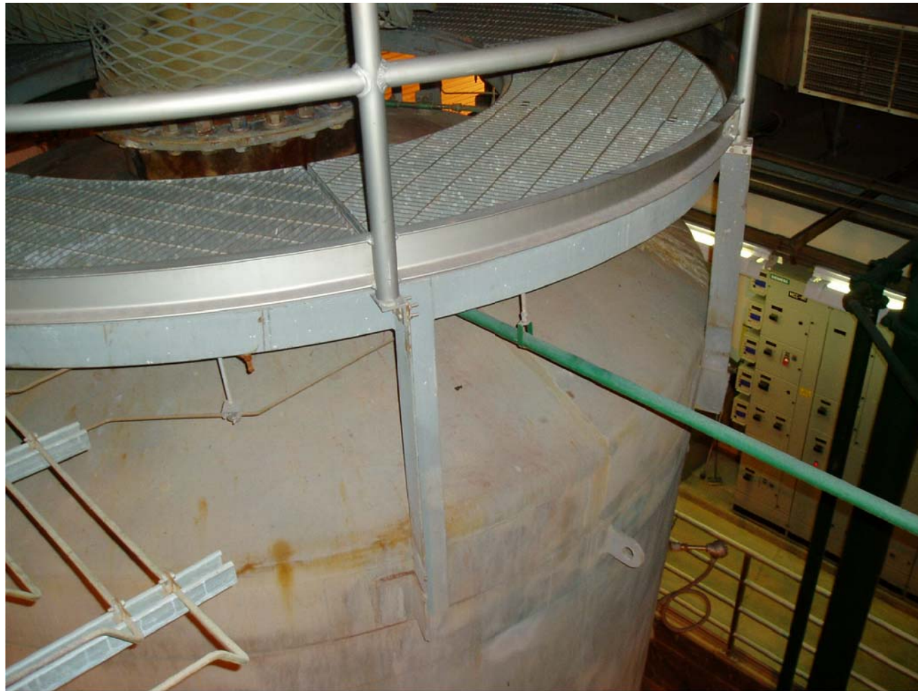
UPPER PLATFORM SUPPORT
