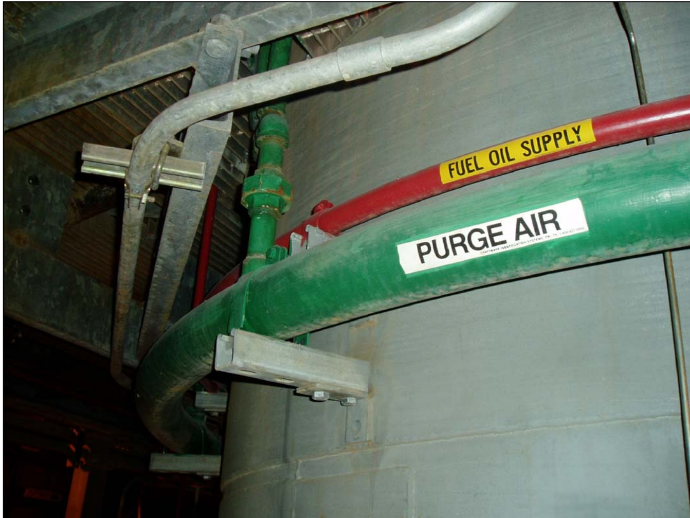
TYPICAL WELDED SUPPORTS LOWER BELLY BAND
