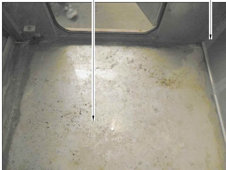
3 EXHIBIT PHOTO - COMPARTMENT #2 HX OUTSIDE AIR
