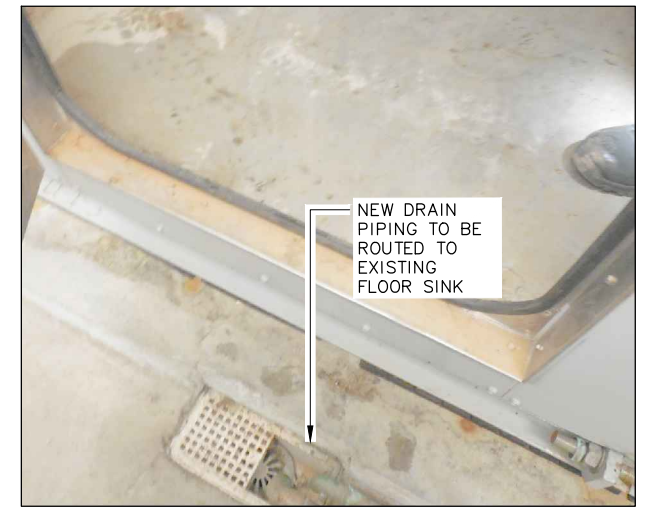
2 EXHIBIT PHOTO - EXISTING FLOOR SINK COMPARTMENT #2 SCALE: NOT TO SCALE
