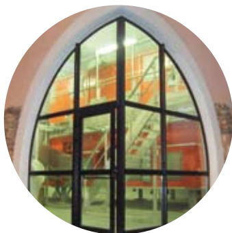
2006: Draguignan Wastewater Treatment Plant, France 1,638 tons dry solids per year
