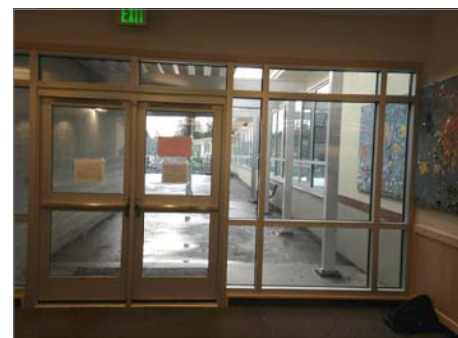
5 Window and door leading to playground from Commons Area.
