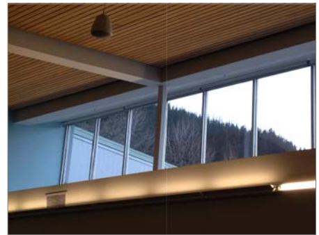
3 Upper Windows in Commons Area facing NW.
