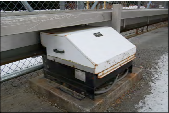
EXIST. SLIDING GATE OPERATOR
