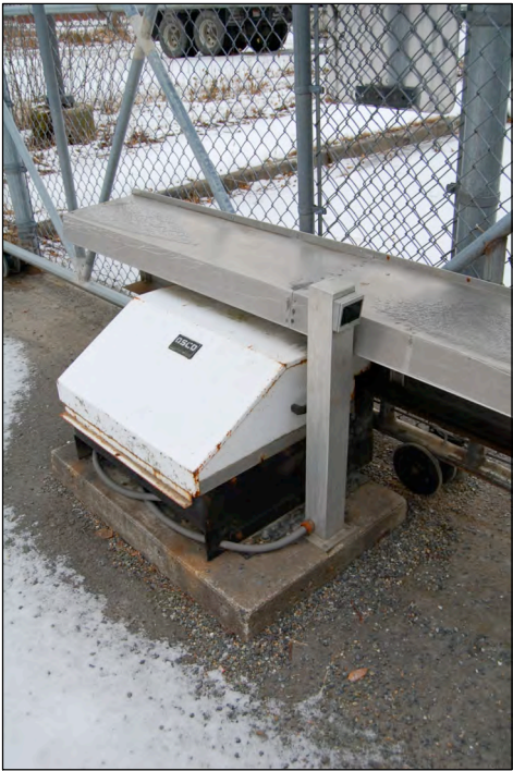
EXIST. SLIDING GATE OPERATOR
