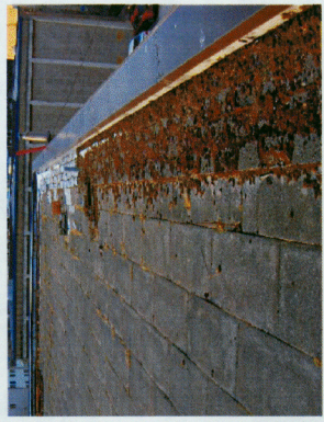
B-2 OVERALL VIEW
