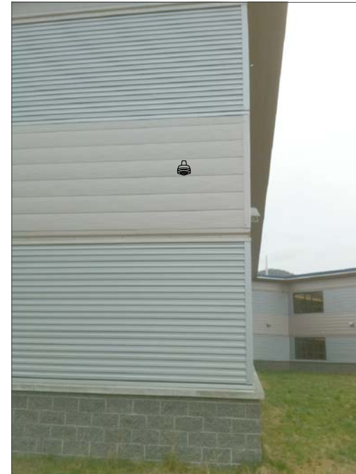
CT7- WALL MOUNT, FEED FROM ABOVE SUSPENDED CEILING IN CLASSROOM. ROUTE ABOVE SUSPENDED CEILING TO IT CABINET.
