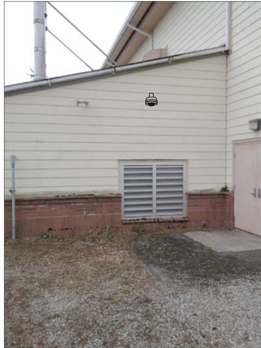
CR14- WALL MOUNT, FEED FROM ABOVE CEILING. SURFACE MOUNT CONDUIT IN MECHANICAL SPACES TO IT CABINET ON SECOND FLOOR.
