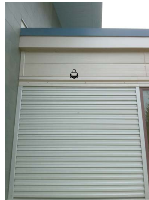
CT11- EXTERIOR WALL MOUNT ABOVE INTERIOR CEILING, FEED FROM ABOVE CEILING. ROUTE ABOVE SUSPENDED CEILING TO IT CABINET.
