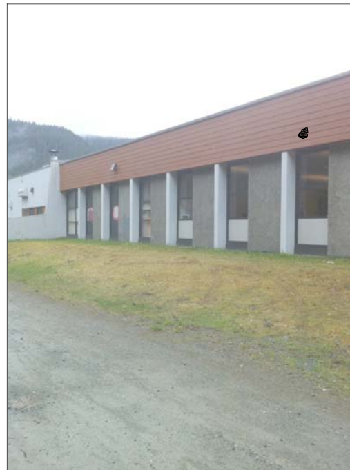
CF7c- WALL MOUNT TO HARDI PLANK, FEED FROM ABOVE SUSPENDED CEILING IN CLASSROOM. SUSPENDED CEILING AT 9'-10".
