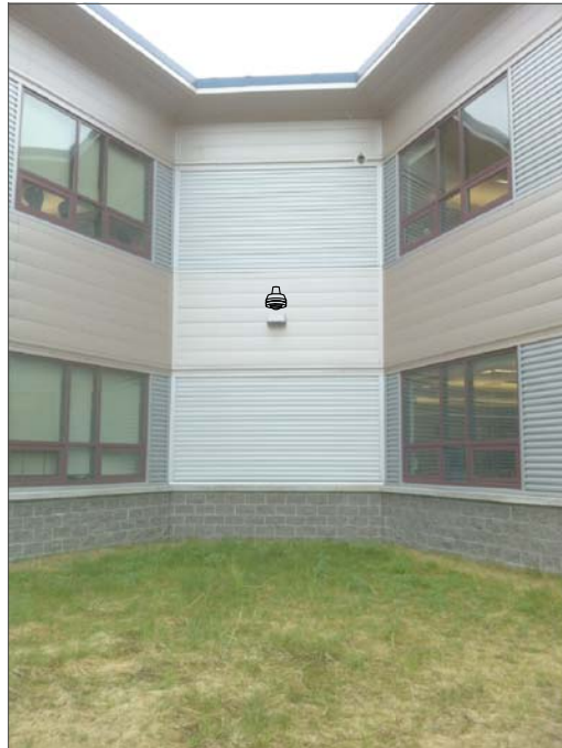
CT6- WALL MOUNT ON SECOND FLOOR EXTERIOR WALL ABOVE CEILING IN STORAGE/PREP ROOM, FEED FROM ABOVE ROOM CEILING. ROUTE ABOVE SUSPENDED CEILING TO IT CABINET.
