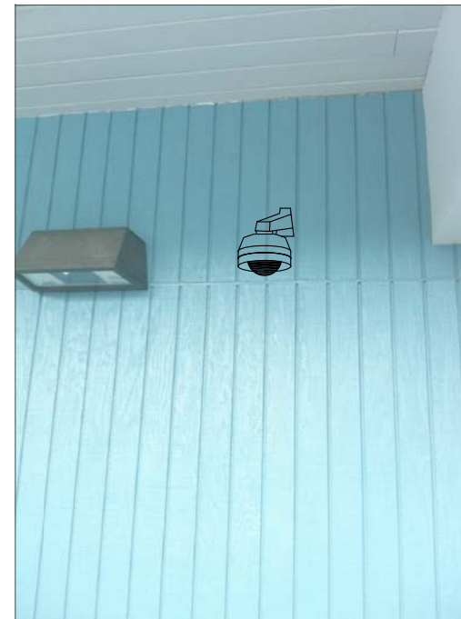
CG13- WALL MOUNT, FEED FROM ABOVE SUSPENDED CEILING IN KITCHEN. SUSPENDED CEILING AT 9'.
