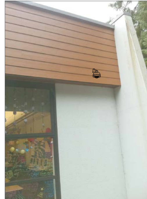
CF10- WALL MOUNT TO HARDI PLANK, FEED FROM ABOVE SUSPENDED CEILING IN CLASSROOM. SUSPENDED CEILING AT 9'-10".
