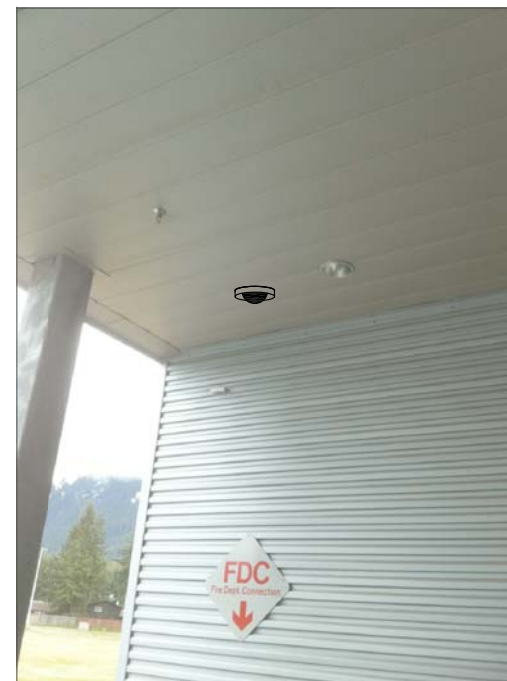
CT15- CEILING MOUNT, FEED FROM SURFACE CONDUIT IN BOILER ROOM. ROUTE CONDUIT TO ABOVE SUSPENDED CEILING IN CORRIDOR THEN TO IT CABINET.
