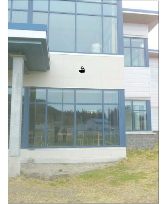
CT4- WALL MOUNT, FEED FROM ABOVE INTERIOR SUSPENDED CEILING. ROUTE ABOVE SUSPENDED CEILING TO IT CABINET.
