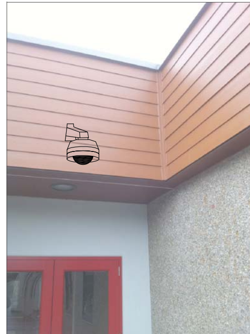
CF3- WALL MOUNT TO HARDI PLANK. FEED FROM ABOVE SUSPENDED CEILING IN HALL THROUGH SOFFIT SPACE THEN TO CAMERA. SUSPENDED CEILING AT 9'-10".
