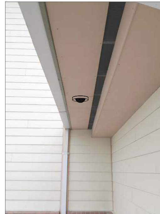
CR11- CEILING MOUNT IN SOFFIT, FEED FROM HALL ACROSS KITCHEN ABOVE CEILING THEN ACROSS TABLE STORAGE ROOMS ABOVE CEILING. ROUTE FROM HALL CEILING TO IT CABINET ON SECOND FLOOR. NIPPLE THROUGH SECOND FLOOR TO CABINET.
