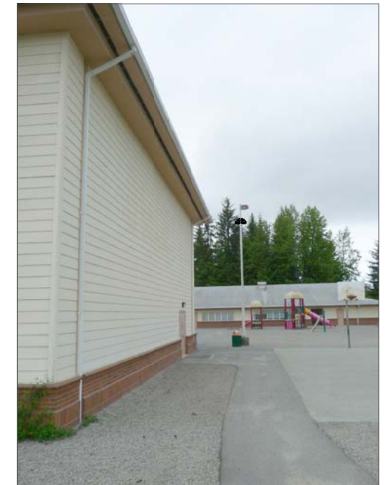
CR12, 13- MOUNT TO POLE. ROUTE CABLES DOWN INSIDE OF POLE, THEN LB OUTSIDE OF POLE AND DOWN UNDERGROUND TO BUILDING. (4)
