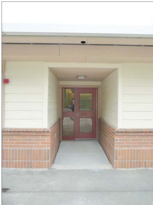
CF4a- CEILING MOUNT IN SOFFIT FEED FROM ABOVE CORRIDOR CEILING THROUGH SOFFIT. ROUTE TO NEAREST CLASSROOM ABOVE SUSPENDED CEILING THEN DOWN CLASSROOM WALL IN WIREMOLD 500 TO EXISTING RACEWAY THEN VIA EXISTING RACEWAY TO IT CABINET.
