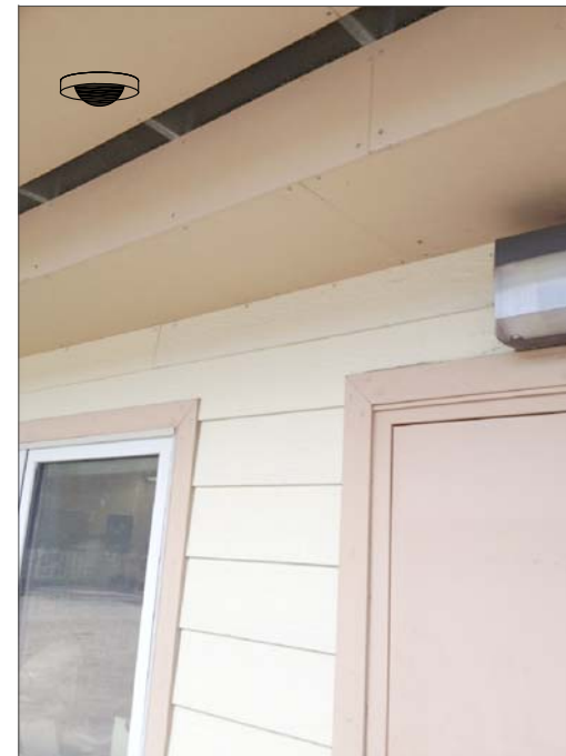
CR6- MOUNT IN SOFFIT, FEED FROM ABOVE SUSPENDED CEILING IN HALLWAY THROUGH SOFFIT TO CAMERA. ROUTE TO NEAREST CLASSROOM ABOVE SUSPENDED CEILING THEN DOWN CLASSROOM WALL IN WIREMOLD 500 TO EXISTING RACEWAY THEN VIA EXISTING RACEWAY TO IT CABINET.
