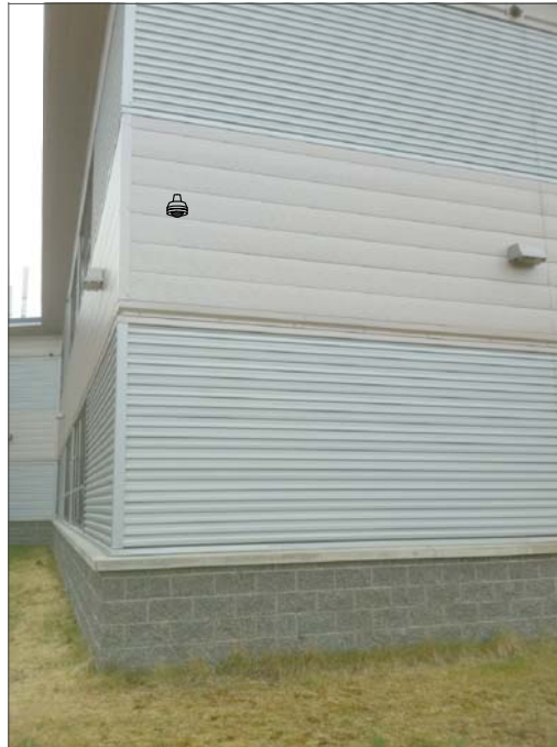
CT5- WALL MOUNT, FEED FROM ABOVE SUSPENDED CEILING IN CLASSROOM. ROUTE ABOVE SUSPENDED CEILING TO IT CABINET.
