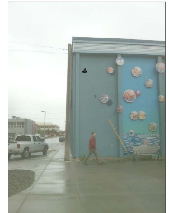
CHB14- WALL MOUNT UNDER EAVE. SURFACE MOUNT UNDER METAL EAVE OVER ENTRANCE THEN DOWN CORNER OF COLUMN TO UNDER ENTRY ROOF THEN BEHIND FASCIA TO ABOVE ADMINISTRATION OFFICE'S SUSPENDED CEILING.
