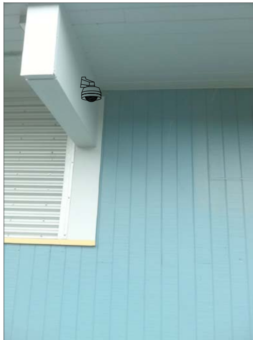
CG12- WALL MOUNT ON RIGHT SIDE OF BEAM. DRILL THROUGH BEAM SURFACE MOUNT CONDUIT TO BACK SIDE OF IT CABINET, FEED THROUGH WALL INTO CABINET. (5)
