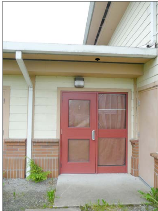
CR2- CEILING MOUNT, FEED THROUGH SOFFIT TO WIREMOLD J-BOX, THEN IN WIREMOLD 500 DOWN INTERIOR OF WALL TO EXISTING SURFACE RACEWAY, THEN VIA RACEWAY TO IT CABINET. (4)
