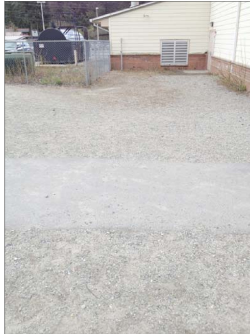
ASPHALT PATH- ROUTING: CUT ASPHALT PATH TO FEED CR12 & 13. PATCH CUT PAVEMENT.
