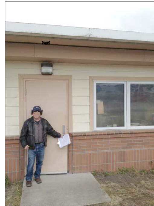
CR3- CEILING MOUNT, FEED THROUGH SOFFIT TO WIREMOLD J-BOX, THEN IN WIREMOLD 500 DOWN INTERIOR OF WALL TO EXISTING SURFACE RACEWAY, THEN VIA RACEWAY TO IT CABINET.
