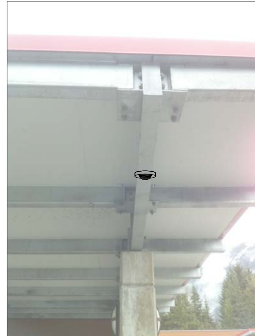
CF17- MOUNTED ON COVERED WALKWAY STRUCTURE. MOUNT SAME AS CF16, FEED FROM ABOVE CEILING PANELS IN ENTRY. THEN FROM ABOVE SUSPENDED CEILING INSIDE. (7)
