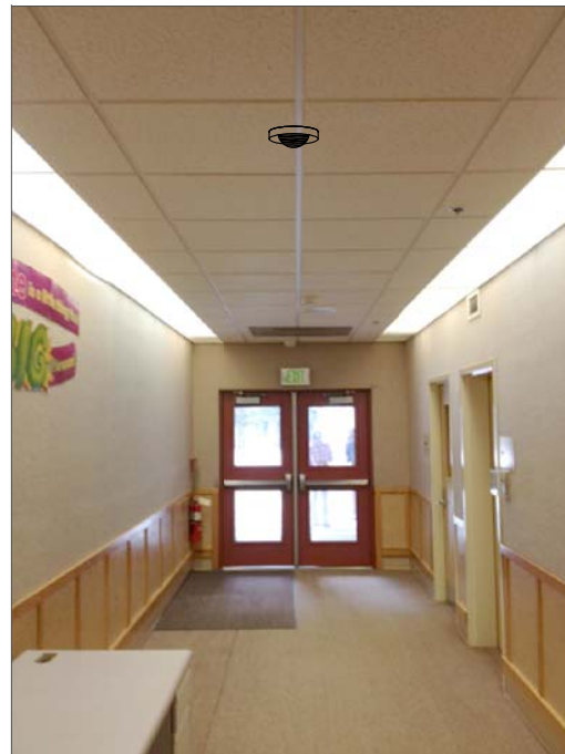
CR5- INTERIOR CAMERA, MOUNT TO SUSPENDED CEILING, FEED FROM ABOVE CEILING. ROUTE TO NEAREST CLASSROOM ABOVE SUSPENDED CEILING THEN DOWN CLASSROOM WALL IN WIREMOLD 500 TO EXISTING RACEWAY THEN VIA EXISTING RACEWAY TO IT CABINET.
