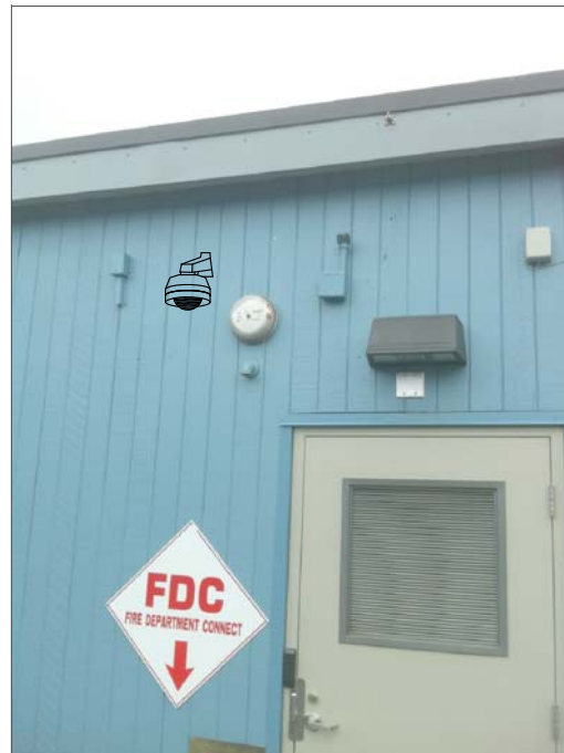
CG12a- WALL MOUNT FEED FROM INSIDE BOILER ROOM WITH SURFACE MOUNT CONDUIT. ROUTE TO NEAREST SWITCH IN CLASSROOM ACROSS HALL FROM BOILER ROOM.
