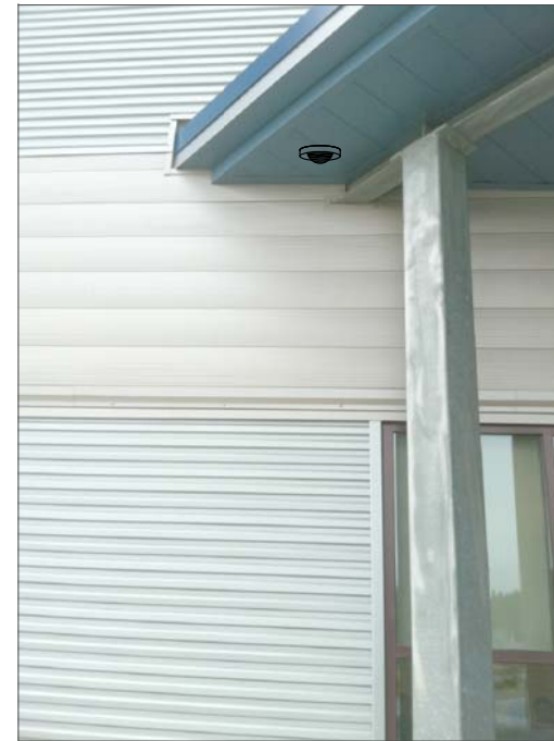
CT3- CEILING MOUNT, FEED FROM ABOVE SOFFIT METAL INTO SPACE ABOVE SUSPENDED CEILING. THEN ABOVE SUSPENDED CEILING TO IT CABINET.
