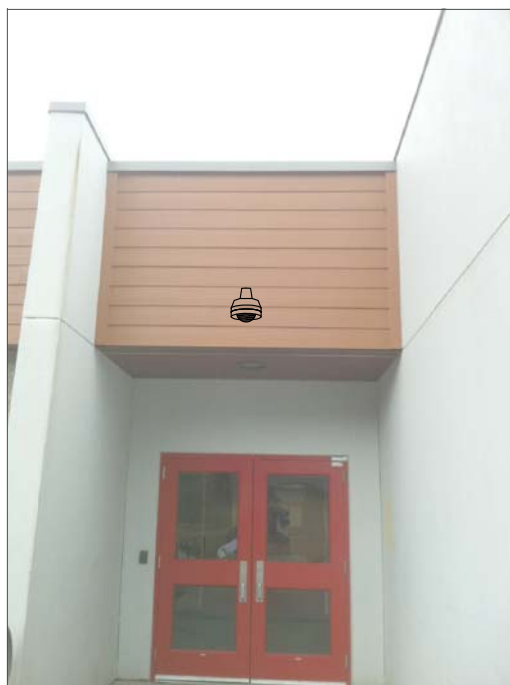
CF6- WALL MOUNT TO HARDI PLANK. FEED FROM ABOVE SUSPENDED CEILING IN HALL, THROUGH SOFFIT SPACE THEN TO CAMERA. SUSPENDED CEILING AT 9'-10".
