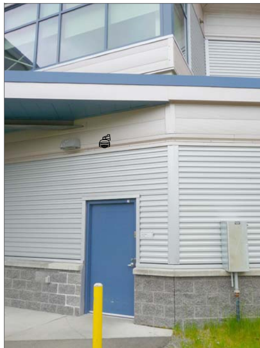
CT10- WALL MOUNT, FEED FROM SUSPENDED CEILING ABOVE CEILING. ROUTE ABOVE SUSPENDED CEILING TO IT CABINET.
