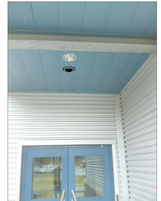
CT16- CEILING MOUNT, FEED FROM SURFACE CONDUIT IN BOILER ROOM. ROUTE CONDUIT TO ABOVE SUSPENDED CEILING IN CORRIDOR THEN TO IT CABINET.
