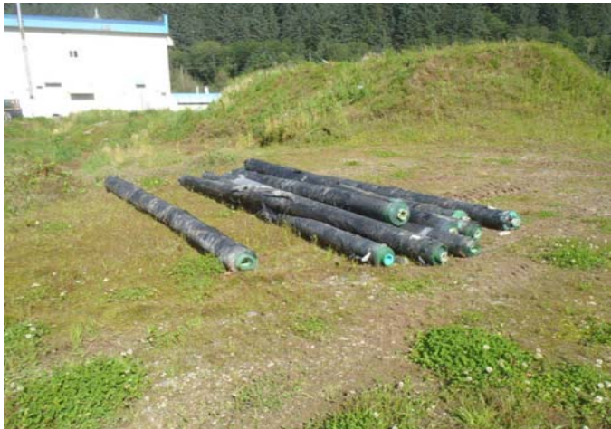
Photo 2: View of Existing Ash Pile With Geotextile Fabric in Foreground
