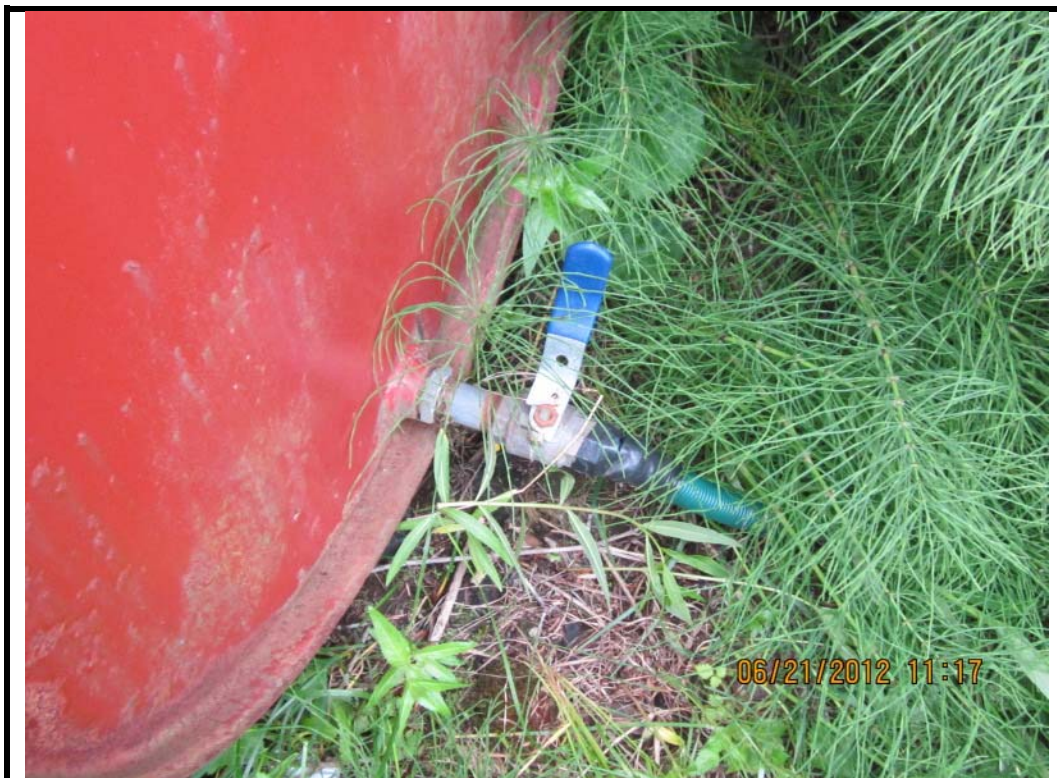
Photo 10: Improper fuel line connection on AST. Area of soil contamination.
