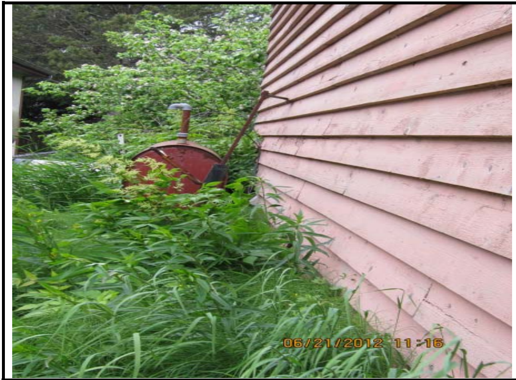
Photo 9: Aboveground fuel storage tank on South side of residence.
