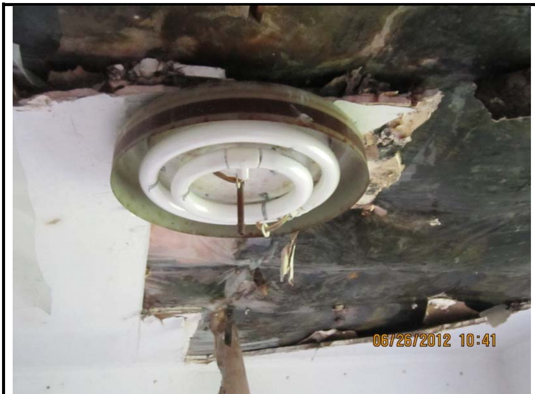
Photo 12: Example of hazardous materials identified inside residence.
