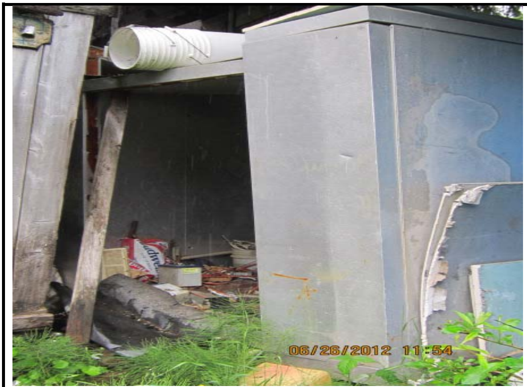
Photo 8: Large shed is partially constructed of old freezer, potential hazmat.
