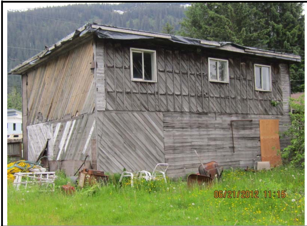
Photo 2: Rear of residence, showing west side.
