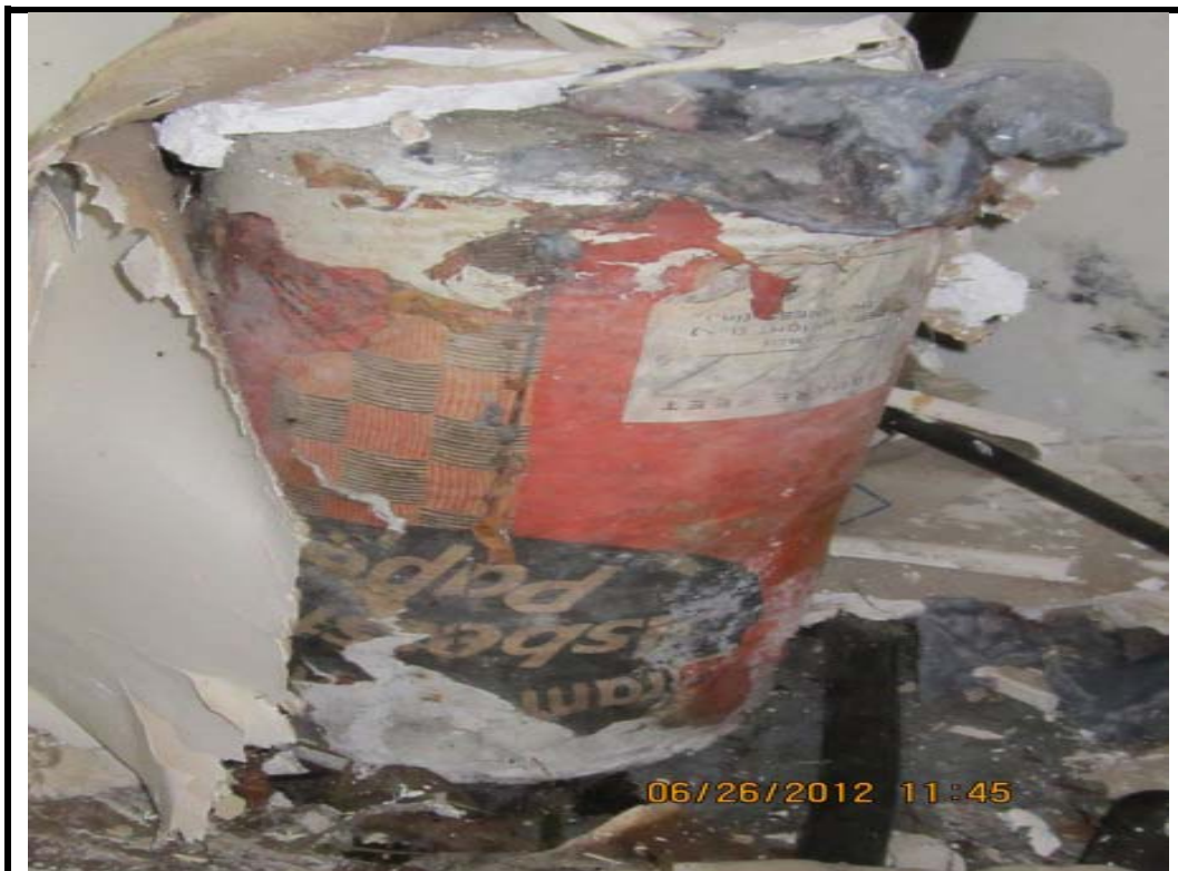
Photo 14: Hazardous material identified in Room 1. Asbestos paper.
